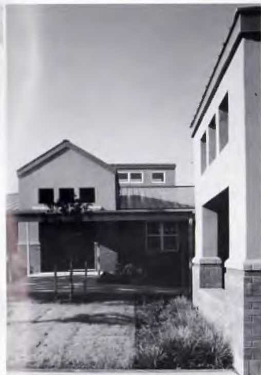
Infant-Parent Training Center: exterior at entry tower
