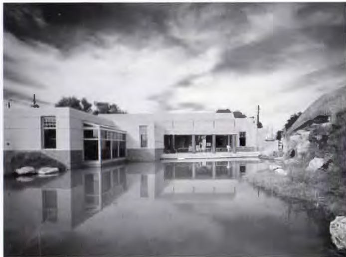
An old sand pit on the site was reclaimed as a water feature.
