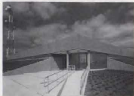
Central Power & Light Energy Control
