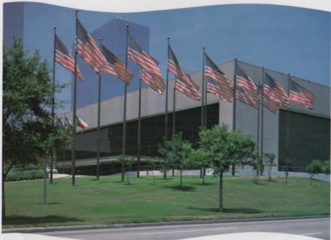
The Summit, Houston, Texas, installed, 1974.
