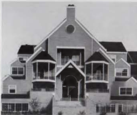
Bryan Place Condominiums, Dallas.
