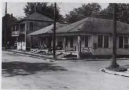
Dilapidated housing in the Fourth Ward.
