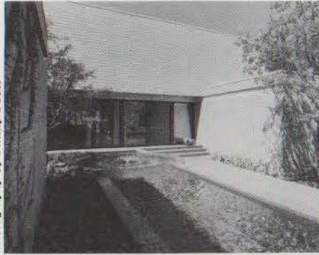
View to entry.
