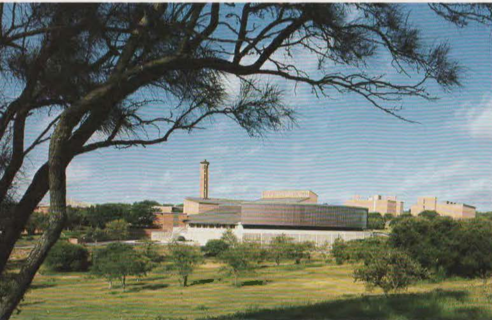
Laurie Auditorium (1970) and Trinity campus, San Antonio, 1950—present (with Bartlett Cocke).
