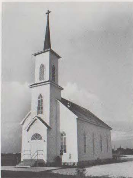
Heritage Presbyterian Church (before).
