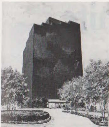
Petro-Lewis Tower, Houston.
