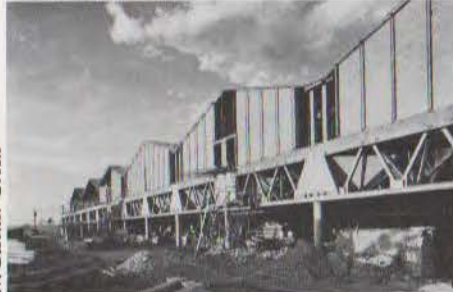
Texas Instruments under construction.
