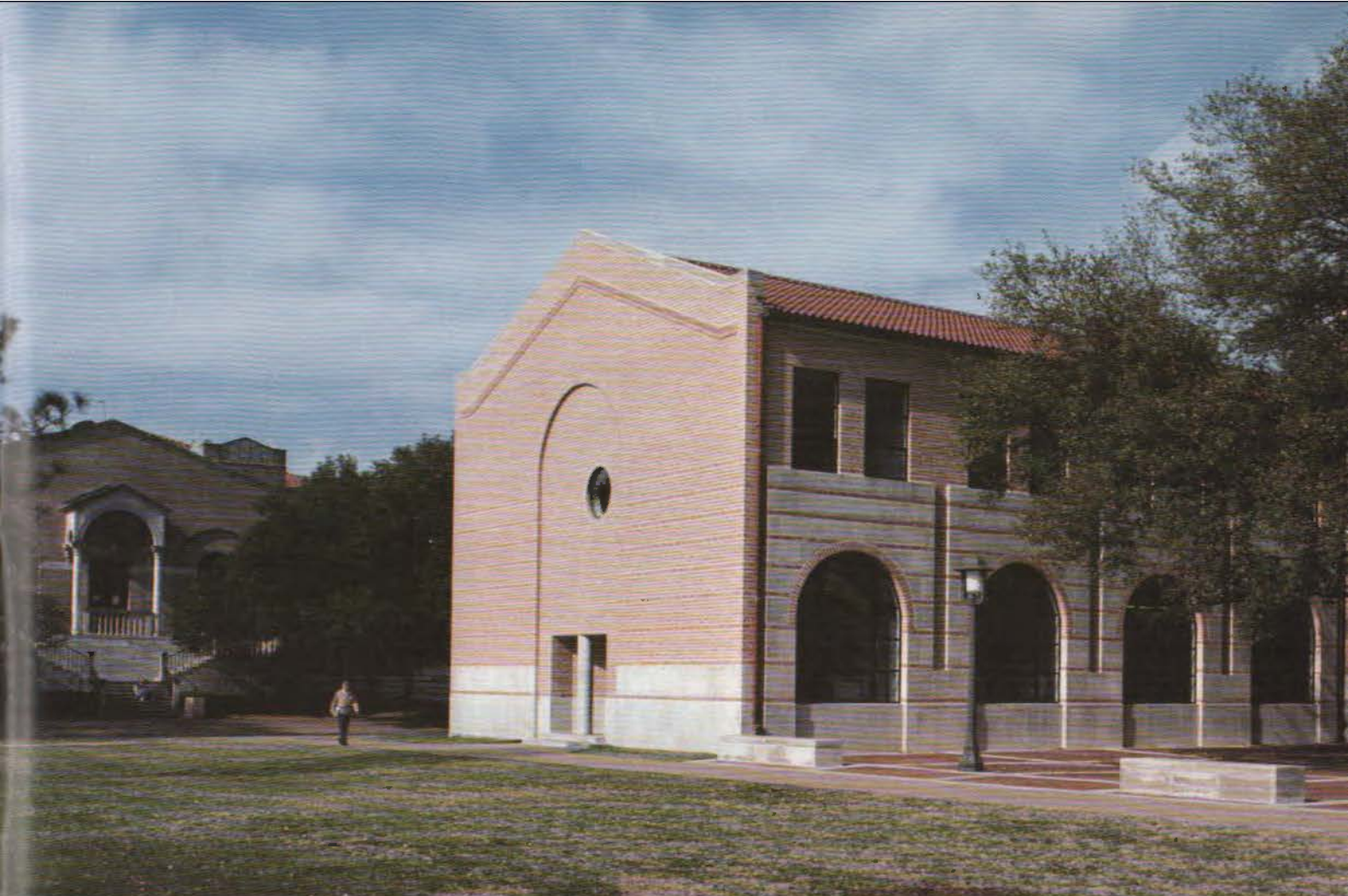
Addition to Anderson Hall, Rice University School of Architecture, James Stirling, Michael Wilford & Associates, 1981: an amiable dialogue between new and old.
