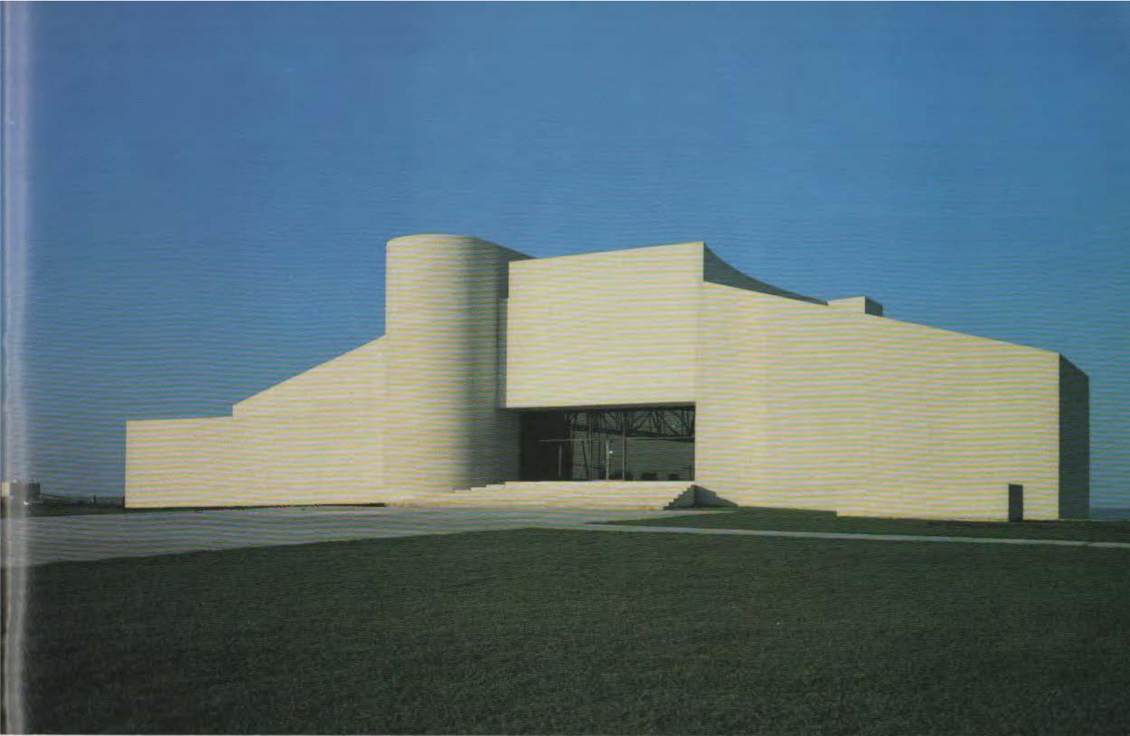
Front facade, Art Museum of South Texas.
