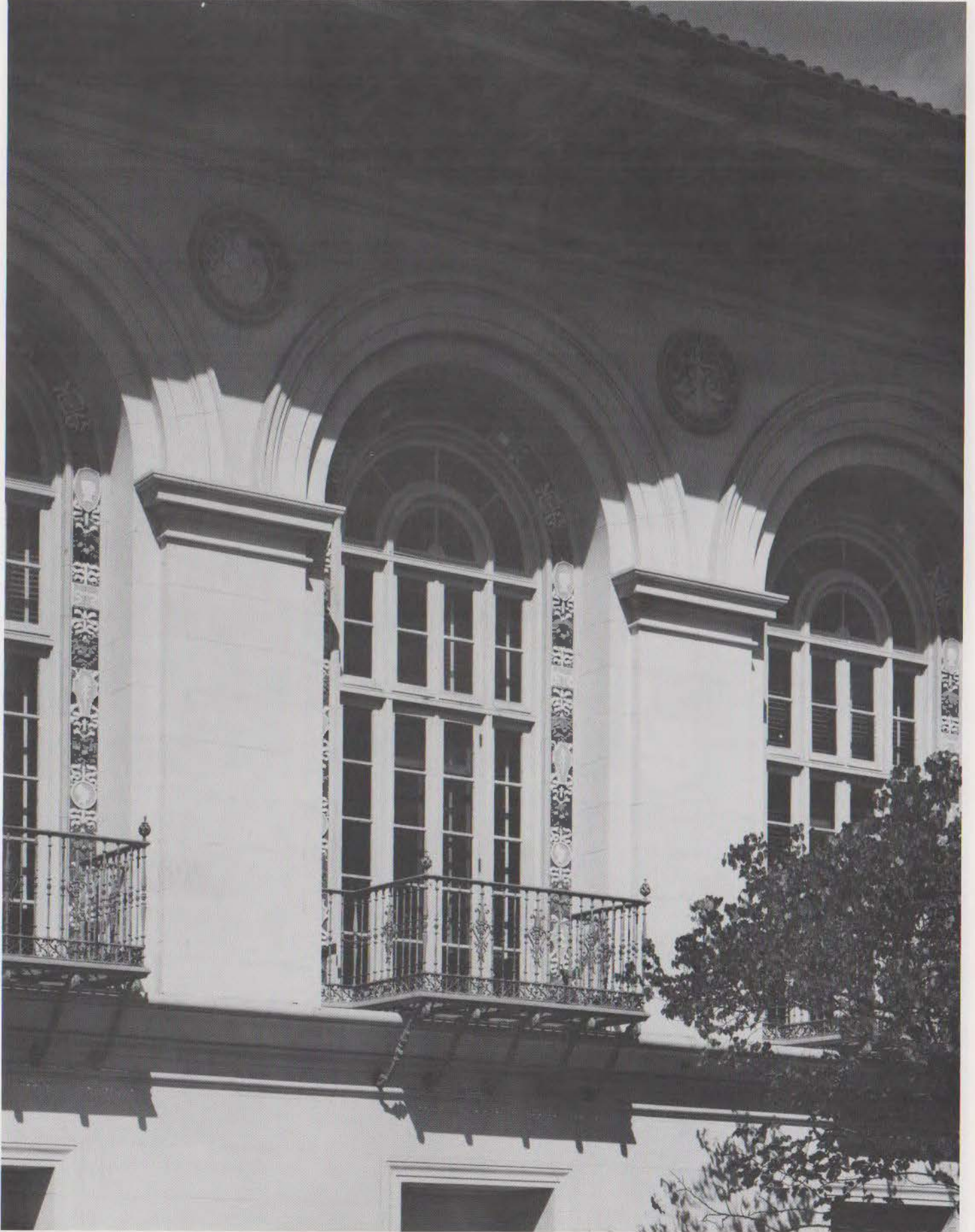
Detail of east facade, Battle Hall, University of Texas at Austin, by Cass Gilbert, 1910.
