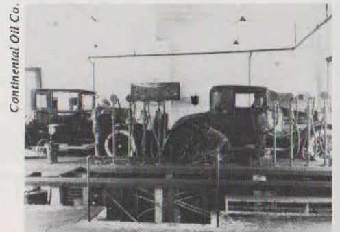
TOP: In 1905, C. H. Laessig (left) developed a technique for gravity-feeding gas to cars at his St. Louis bulk station by attaching a gauge and hose to an old hot water tank (right) filled with gasoline. ABOVE: Addition of pits and lifts helped the "service station" evolve from the "filling station."
