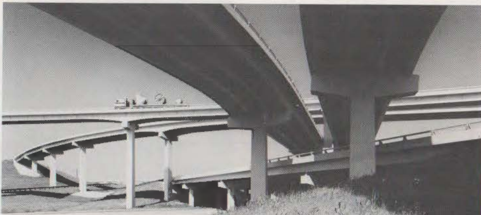
LEFT: I-45/Loop 635 interchange in Dallas. BELOW: I-610/Southwest Freeway interchange in Houston, circa 1964.
