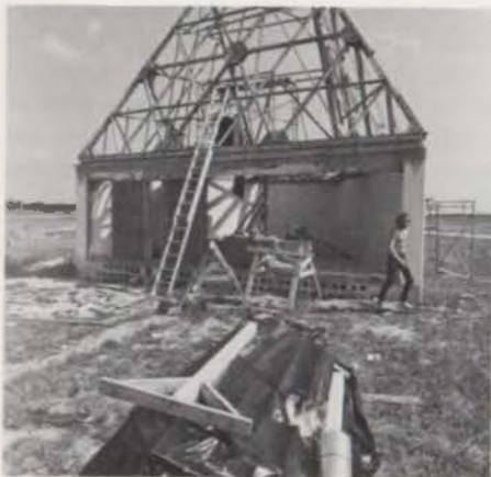
"Greenhouse" under construction.
