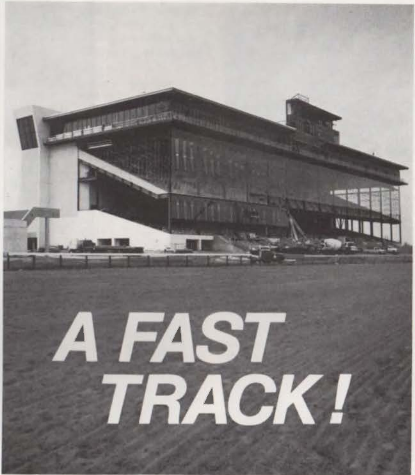
Architect/Engineer: Century A-E Contractor: Henry C. Beck Company
