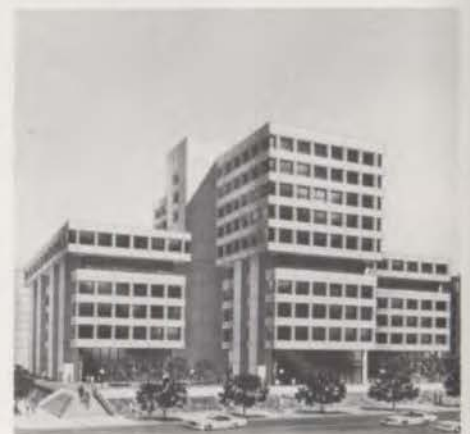
Diagram shows planning concept of "large super-modules of flexible space" permitting low-cost change of function in the Neurosensory Center (rendering) for Baylor Medical School and the Methodist Hospital in Houston. The building is designed to expand horizontally and vertically by 100%.
