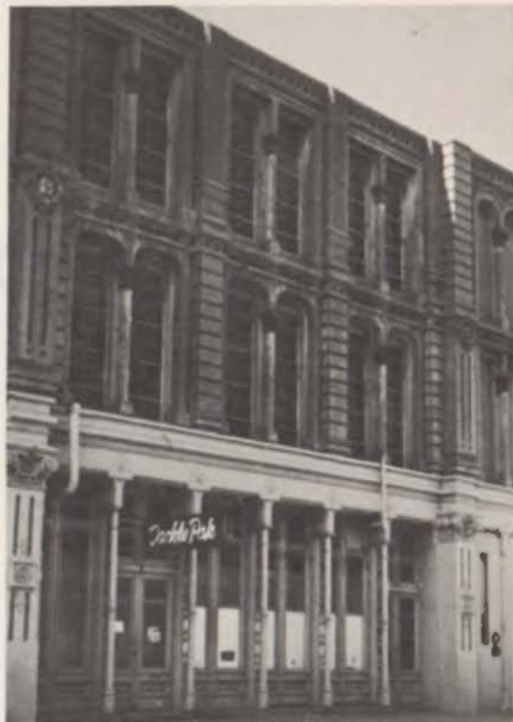
W. L. MOODY BUILDING
