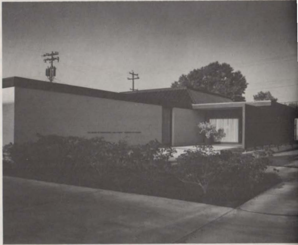
Simplicity of materials and elegance of detail make this an office building that is unobtrusive and welcome in a residential neighborhood.
