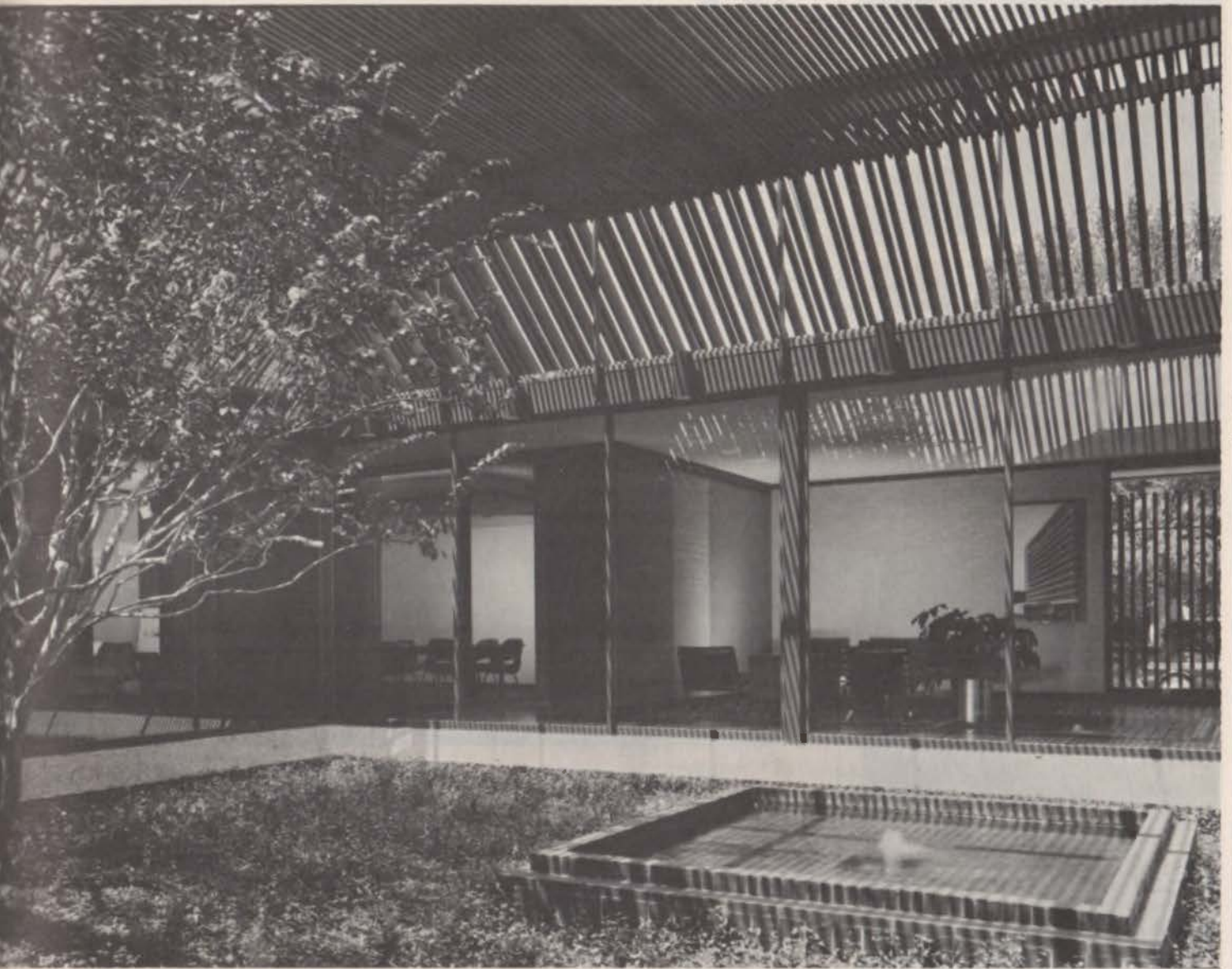
Working spaces are grouped about a courtyard, enclosed overhead by a cable-suspended grillwork of redwood, which helps eliminate glare and heat. The court heightens the sense of designed space and affords a visual relief and variety.
