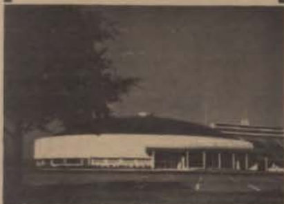
Daniel-Meyer Coliseum, Texas Christian University Fort Worth, Texas Architect: Joseph R. Pelich, A.I.A. After 9 months, no cracks with X-59.
