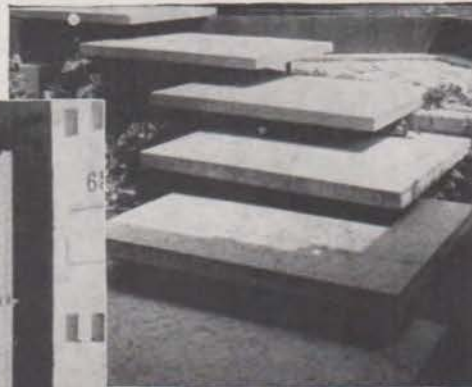
THIN SLAB STEPS OF PRECAST CONCRETE
