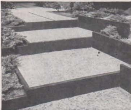
STEPS OF EXPOSED AGGREGATE CONCRETE
