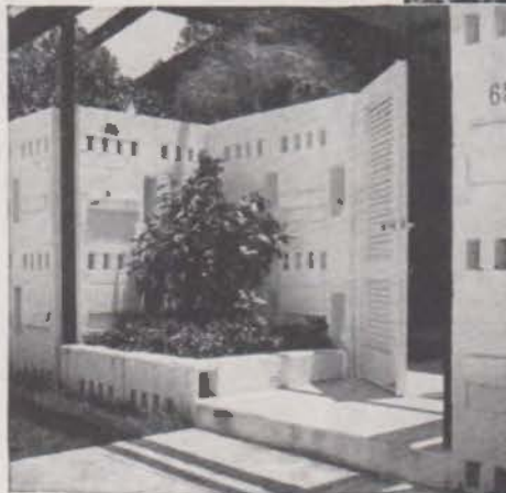
ENTRANCE WALL OF CONCRETE MASONRY
