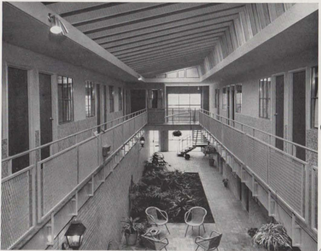
Courtyard of Dallas office building features exposed ceiling joists. Blue Diamond Co. delivered factory-cut Stran-Steel nailable studs and joists to architects and builders Sadler and Armstrong.
