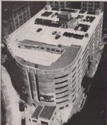
West End Parking Garage, New York City Consulting Engineer: John J. Dwyer, New York City
