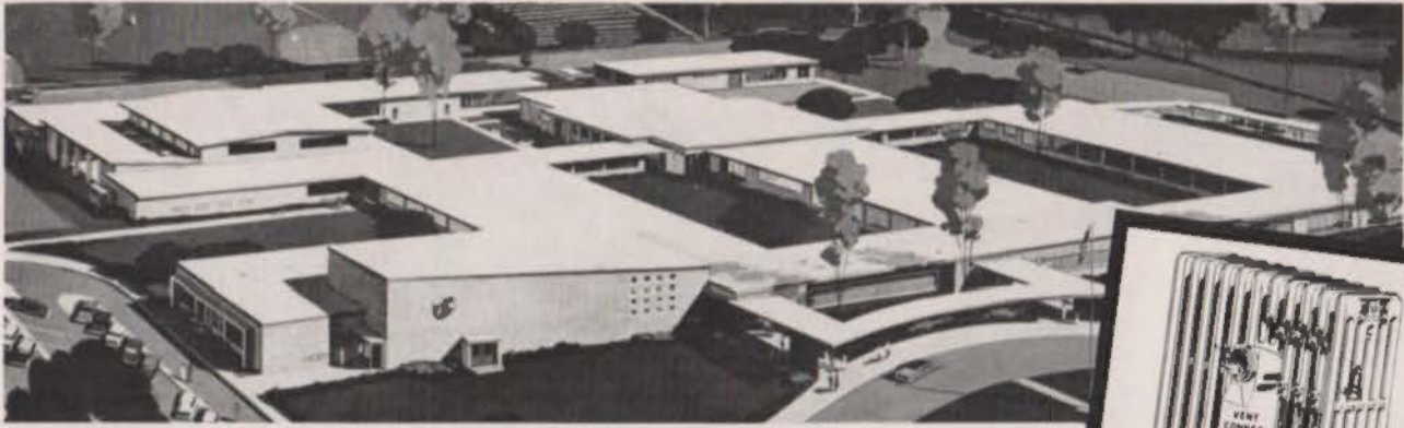
Aldine Senior High School, Aldine, Texas—H. J. Elsik, Superintendent Architects: C. H. Kiefner and Eugene Werlin, Houston Engineer: Raymond L. Jenkins, Houston
