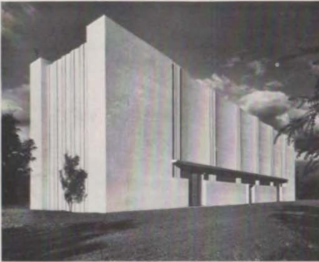
Pumping station, Spokane, Wash.
