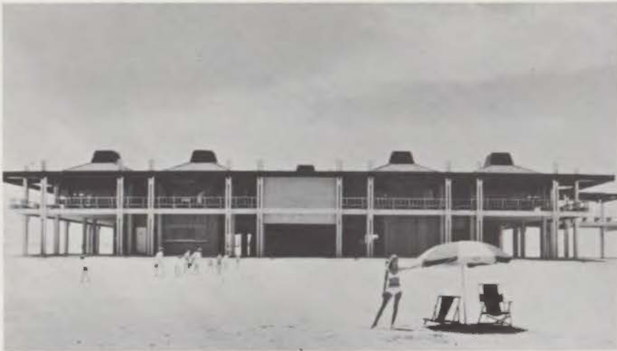
Building A as viewed from the Beach. Note open shelter and concession space at beach level in addition to spacious second level. Flat roof overhang provides additional shaded area. Cupolas maintain a sense of volumetric expansion.
