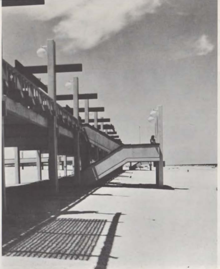
The Boardwalk from beach level in the vicinity of Building A.
