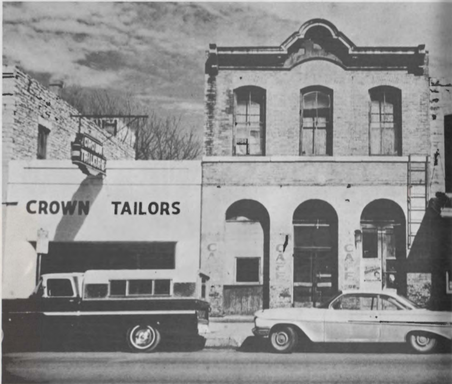
Original Building as purchased in January 1968. Note painted signs, advertising posters, and pass-thru used to serve sidewalk customers.
