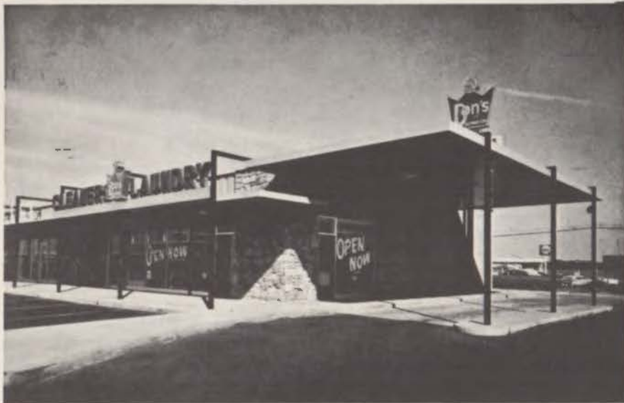
Arapaho Shopping Center utilizes Armco STEELOX Panels for color.
