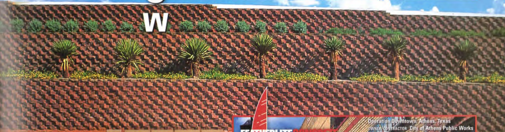
Loop 250 at Lamesa, Midland OWNER/ENGINEER Texas Department of Transportation GENERAL CONTRACTOR Reece Albert, Inc., San Angelo INSTALLER O.A. Moreno & Associates, Inc., Houston
