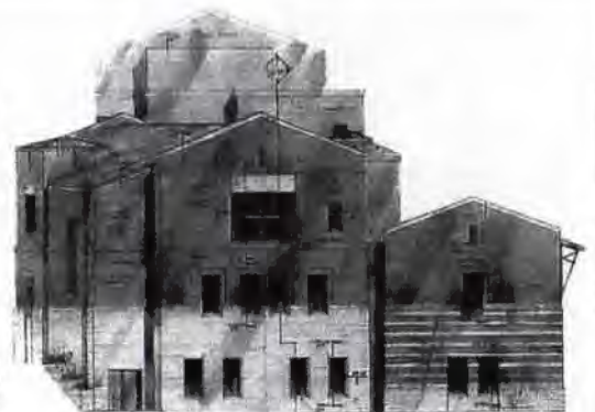
Pictured: Texas School for the Deaf, Austin, Barnes Architects
