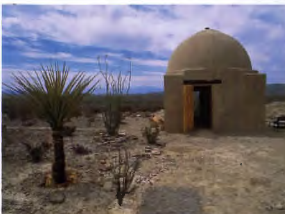
6 Swan says the vaulted roofs are built “with no wood whatsoever, no forms, no centering, no beams.”
