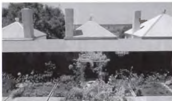
Below left: Metal roofs and site-built caliche blocks provided the primary building materials.
