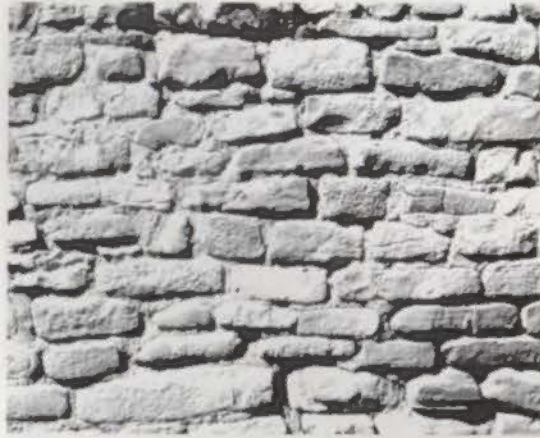
Left: Masonry at Mesa Verde is made from uniform, square stone.
