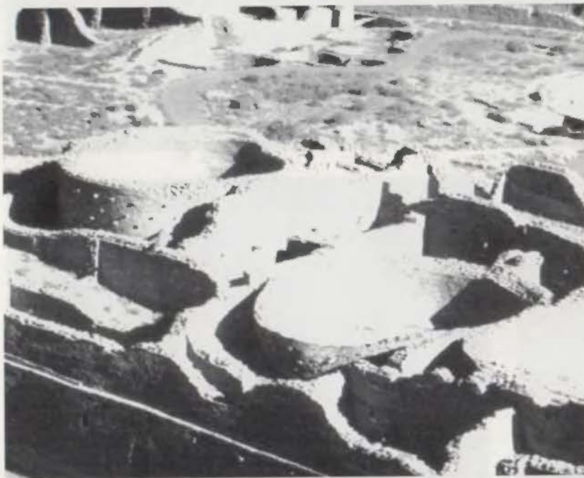
Below: Above-ground kivas at Chetro Ketl were originally enclosed by a rectangular wall configuration, with the poché space backfilled for isolation and silence.
