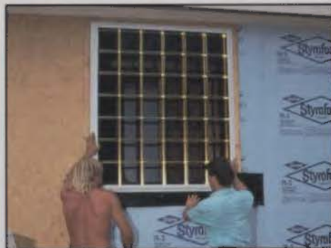
1:30 PM - Install frame
