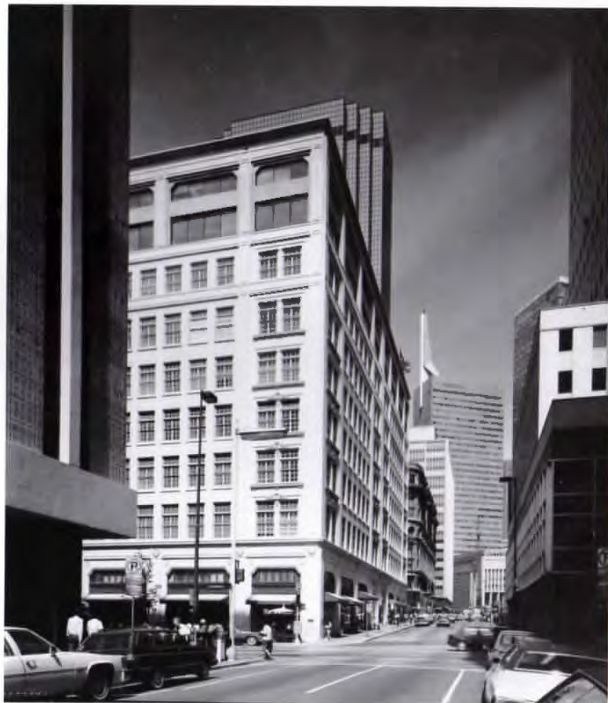
The downtown Neiman Marcus building (1927-28, additions 1940) by Greene, LaRoche & Dahl
