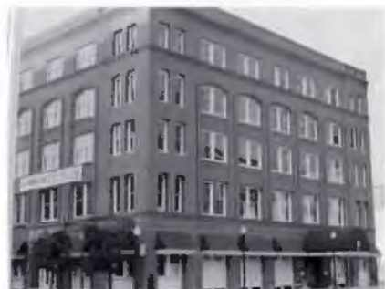
Moline Building —Dallas Built 1905 Renovated 1985 Architect: Corgan & Assoc. Const. Co.: Bartex Inc.
