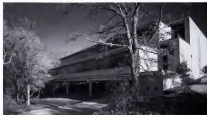
ABOVE: The Oglesby Group made the building present not a three-story mass but a series of receding planes to the neighborhood. Parking is tucked under the building mass. LEFT: Offices enjoy views of the creek.
