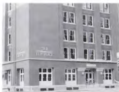
West End One —Dallas Built 1902 Renovated 1986 Architect: Corgan & Assoc. Const. Co.: Julian P. Barry
