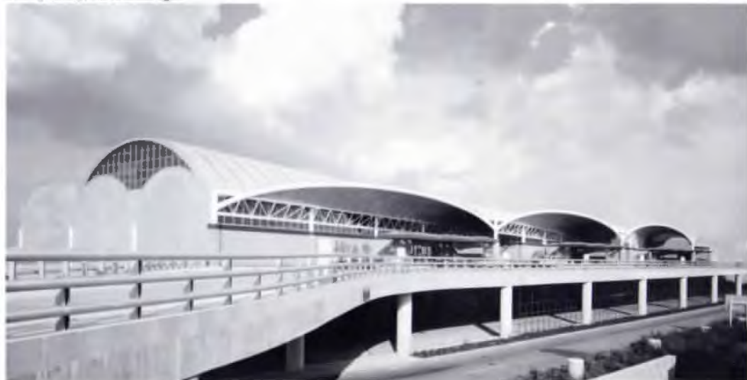
Slicing the arches produced a long, soaring image.
