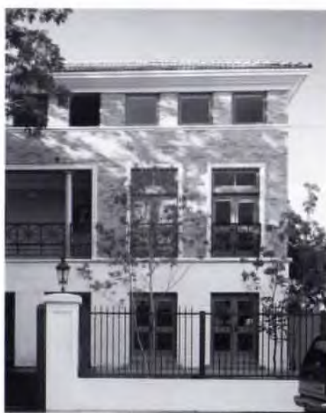
Tile, masonry, brick, columns, and facade arrangement recall Austin's Italianate architecture.
