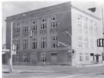
Magnolia Building —Fort Worth Built 1924 Renovated 1986 Architect: Booth & Assoc. Const. Co.: Shoemaker Southwest
