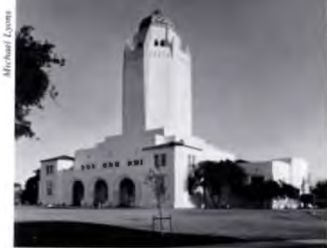
Randolph AFB Administration Building, San Antonio
