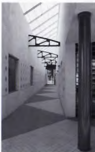
Trusses from an earlier building punctuate the new passageway.
