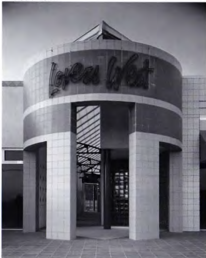
Good, Haas & Fulton gave a strong new identity to a strip that lacked focus.
