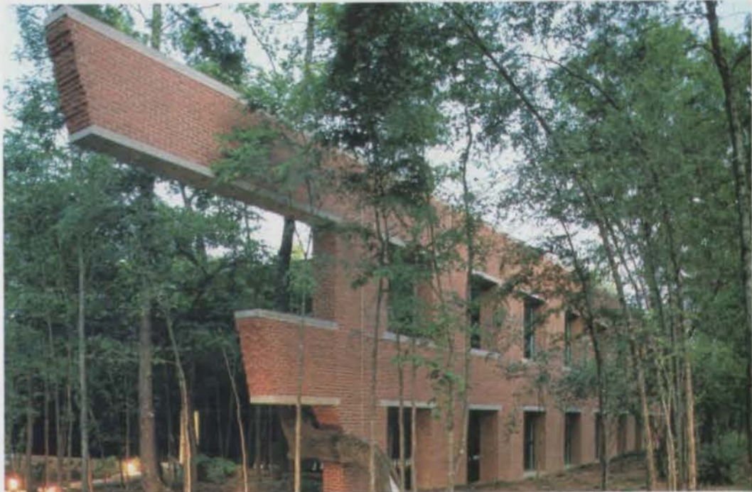
Brick wall "de-constructs" at entrance approach.
