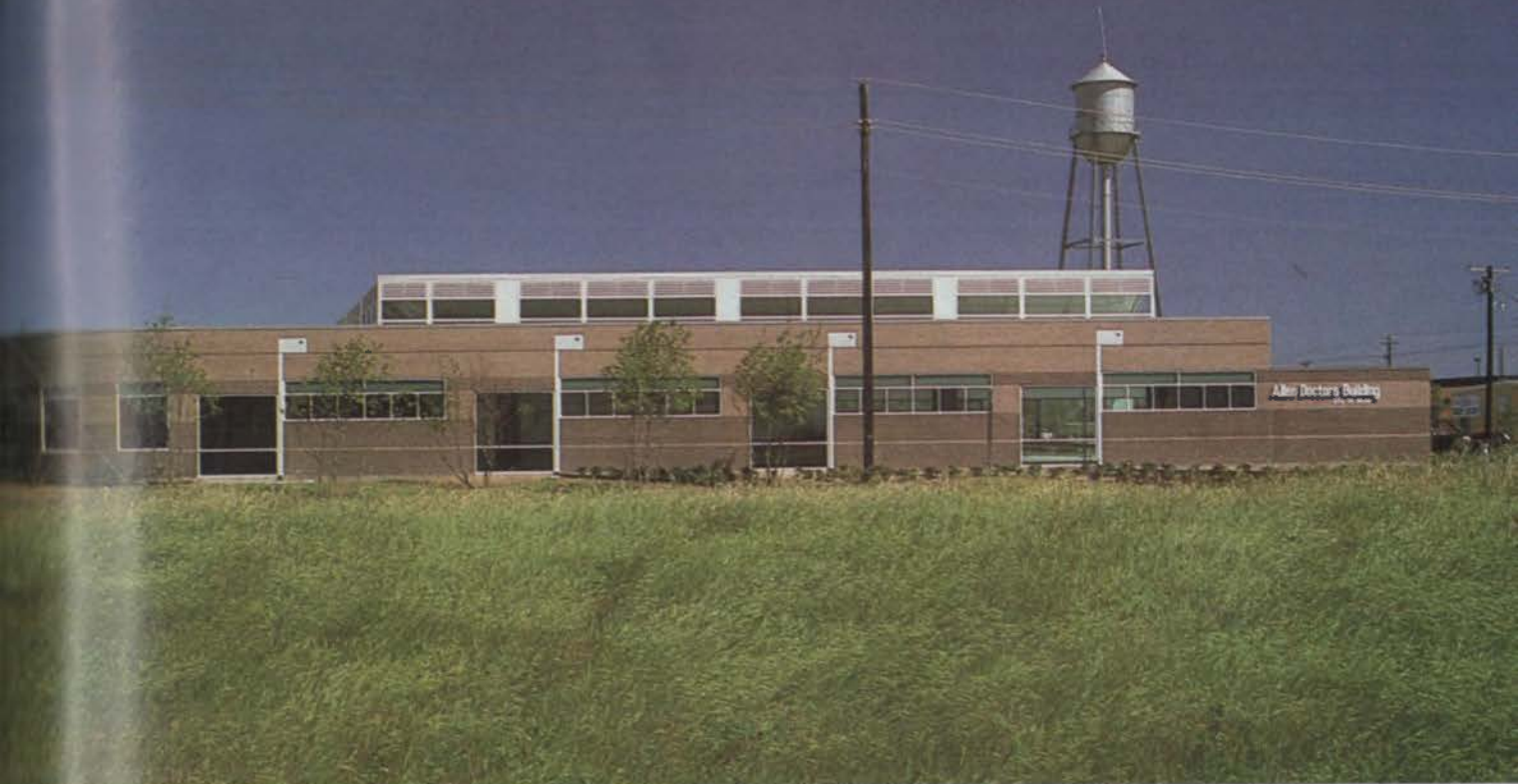
Crisply detailed, the facade is "pinstriped" and uses rainspouts as "doctors' shingles."
