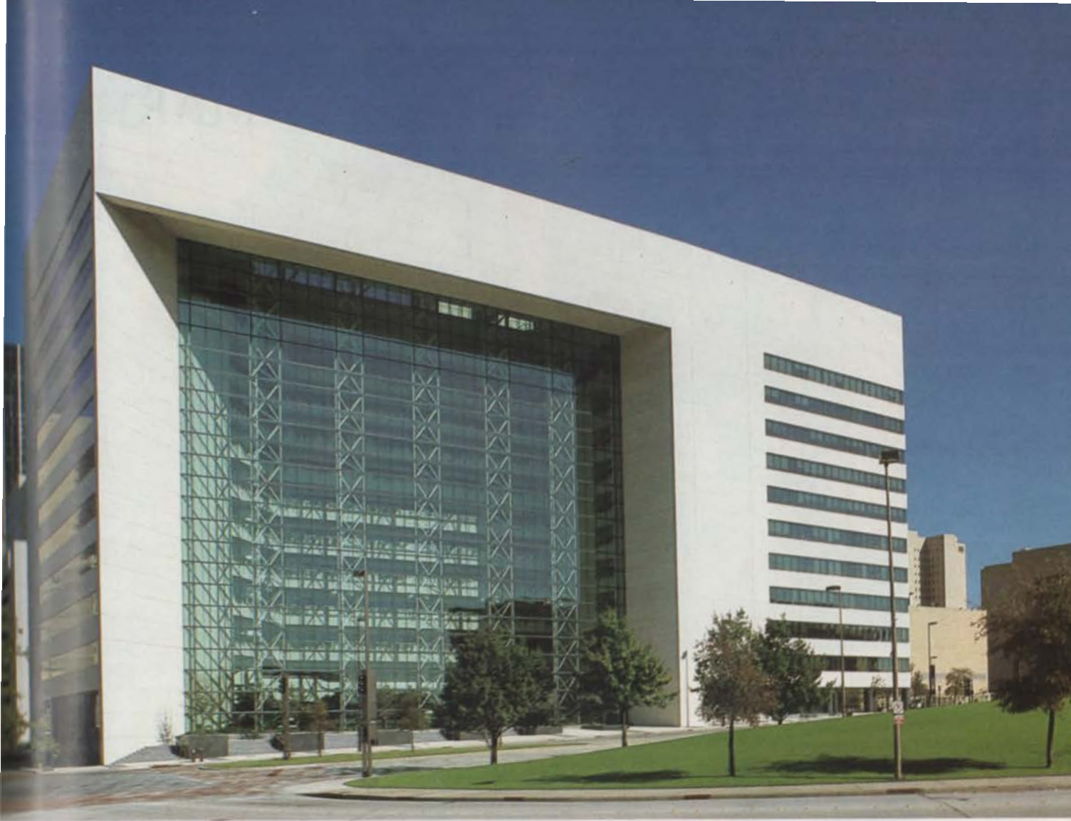
In an area noted for Pei's landmark city hall, the Employers Insurance Building manages not only to be contextual but also to proclaim its own bold presence.
