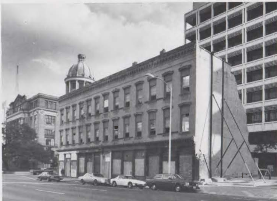
After a long battle to save it, the Pillot building may become a dinner club.
