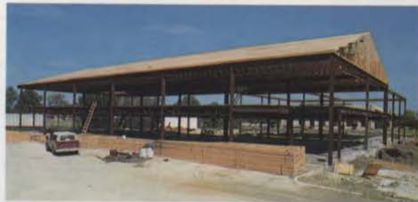
King George Drive Building, Dallas, Texas
