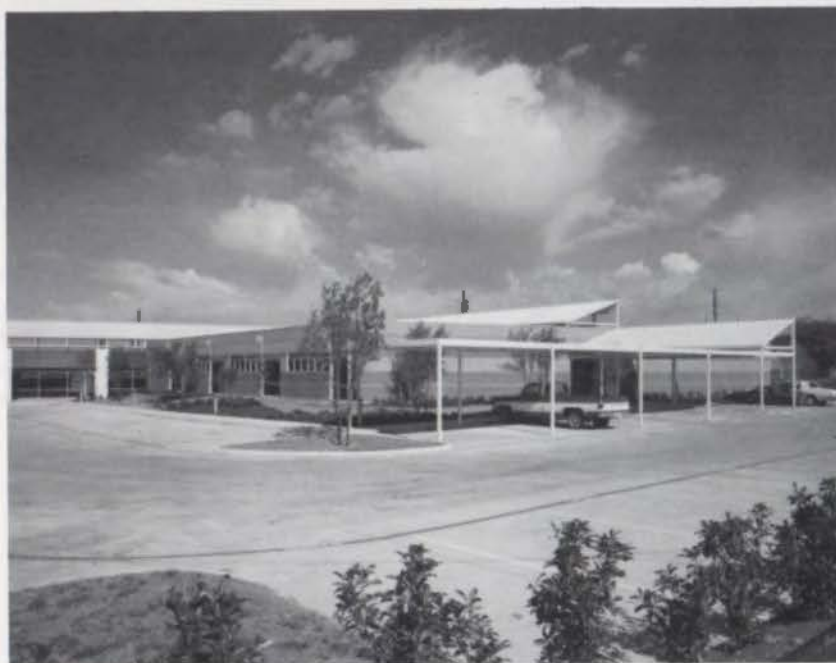
Galleries eliminate space-wasting interior corridors and provide daylight to offices.
