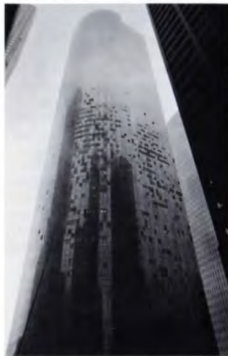
Allied Bank Plaza; Tenneco Building, right.
