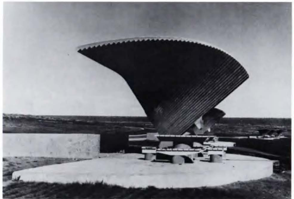
Reinforced concrete shelters at Cherry Creek Recreation Area, by Robert Karl Behrens, Denver, Colorado
