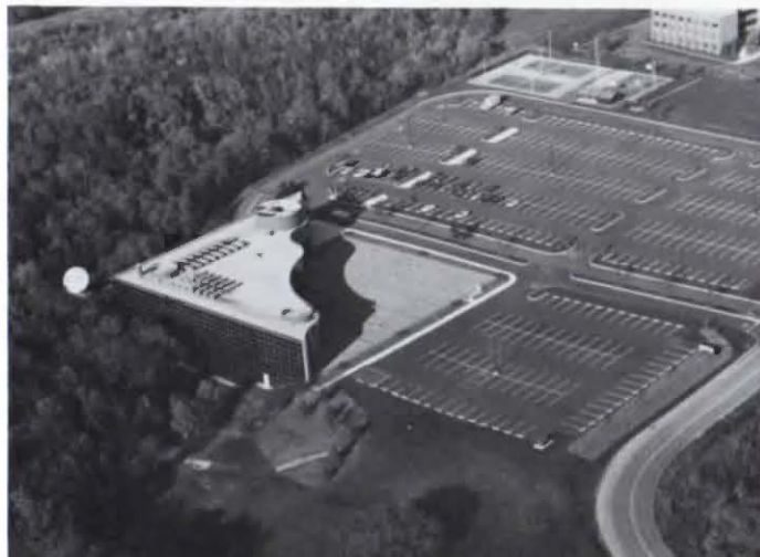
LEFT: Aerial view shows position on ravine. TOP: Wavy facade alludes to undulating treeline. RIGHT: Large-scale metal grid atop below-grade computer room contains pedestal lights that form a pattern of illumination. FAR RIGHT: Glass-block wall admits natural light.
