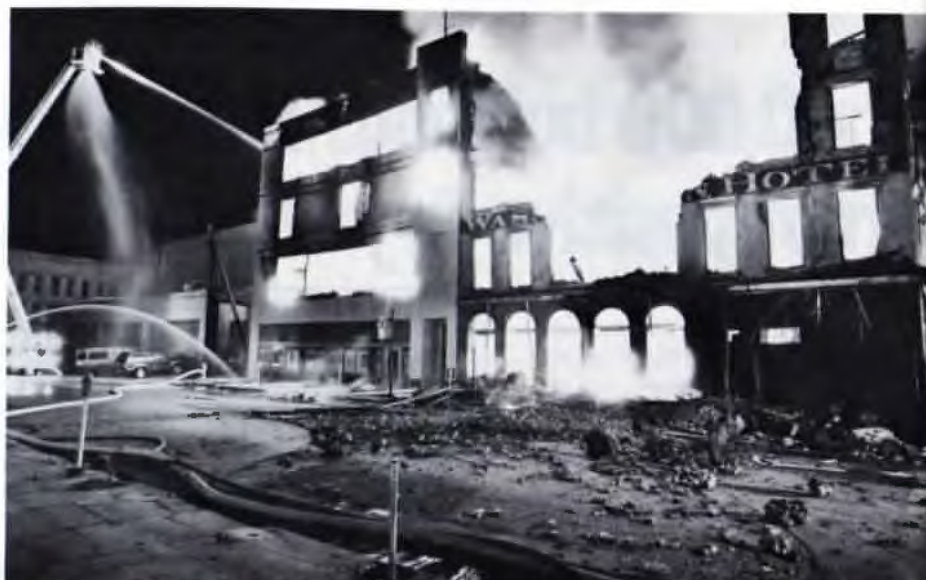
George and Cynthia Mitchell are planning to re-build the fire-damaged Washington Hotel.
