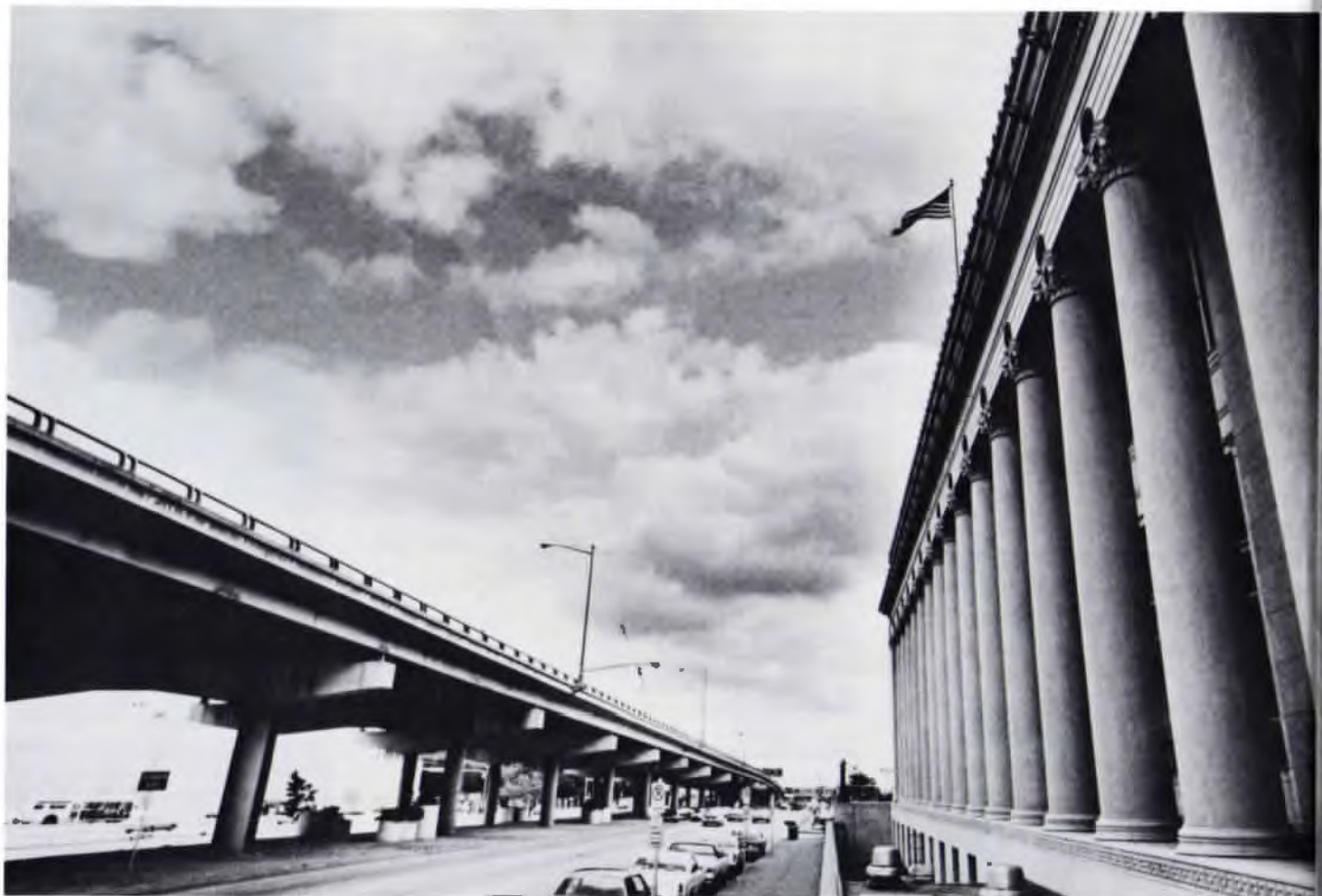
Expansion of I-30 would come within 40 feet of Ft. Worth's historic Main Post Office, right.
