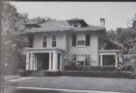
3. Cleveland House, 8 Courtlandt Place, Sanguinet and Staats and A. E. Barnes, architects, 1911.
