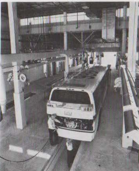
Maintenance stall on outer perimeter.
