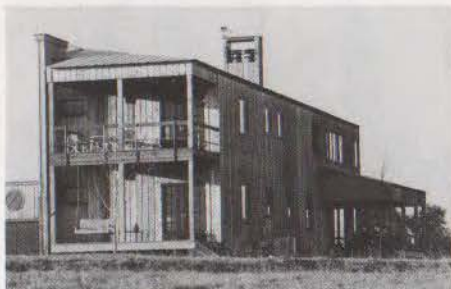
East and north facades.
