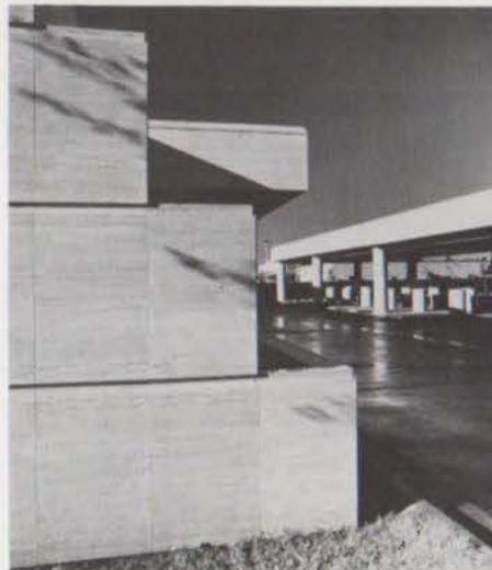
Slipped terraces on drive-in side.
