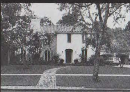
10. Moench House, 13 Courtlandt Place, W. Robert Singleton Associates, architects, 1978.
