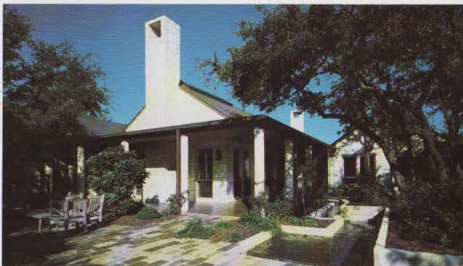
View to library and entry porch.
