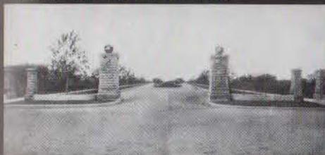
1. East entrance to Courtlandt Boulevard, looking west, showing original piers in place.
