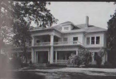
5. Carroll House, 16 Courtlandt Place, J. J. Carroll and the W. T. Carter Lumber and Building Company, designers, 1912.
