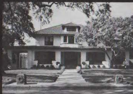
4. Carter House, 18 Courtlandt Place, Olle J. Lorehn, architect, 1912.
