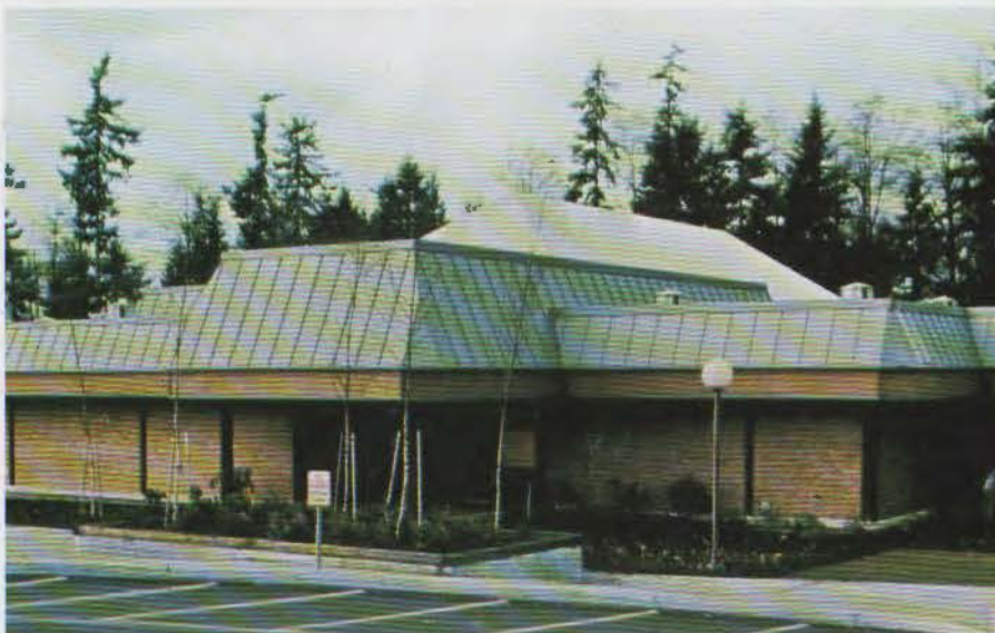
Lynwood Recreation Center, Lynwood, Wash., Architect: ORB Planners & Engineers, Seattle, Wash., Installation: City Heating & Sheet Metal, Inc., Everett, Wash.
