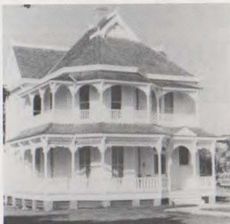
Sidbury House, Corpus Christi.
