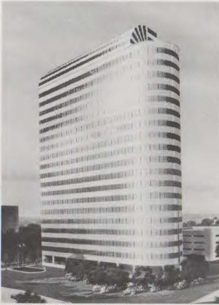
ENSERCH Tower, Houston.
