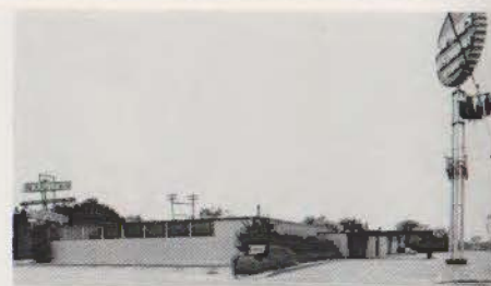
Kaphan's, 7900 S. Main, Claude E. Hooten & H. A. Turner, 1949-50. Early sign is a vestige of time when south Main was the tourist route from San Antonio. Structural bents of entry canopy echo sign form.
