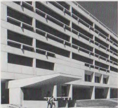
Classroom and office building.
