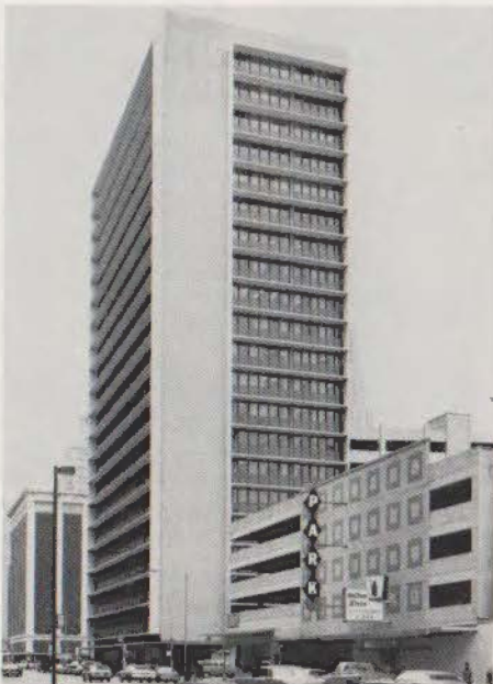
Melrose Building, Walker Ave. and San Jacinto St., Lloyd & Morgan, 1949-52. The essential plan is the L-shape 1920s skyscraper. Advantageous corner office space is curiously given over to the game of vertical vs. horizontal.
