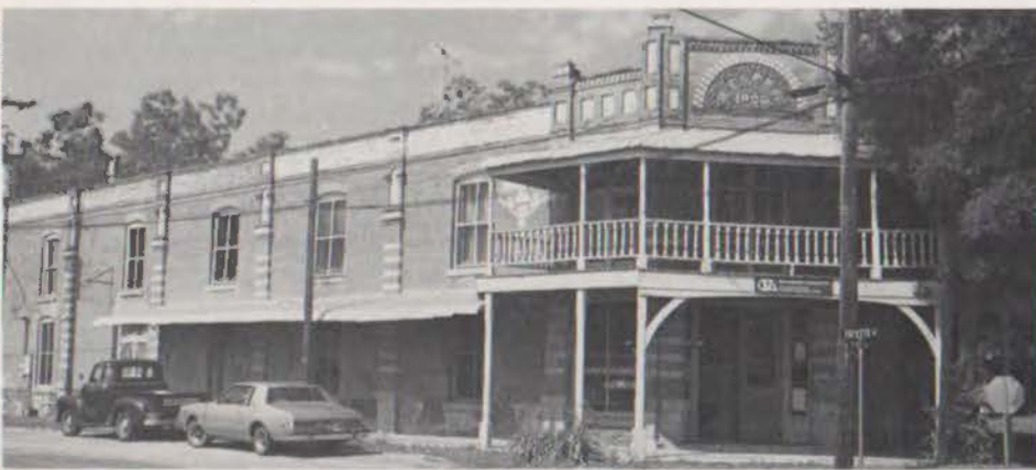
The author's renovated mercantile building on the Fayetteville Square.
