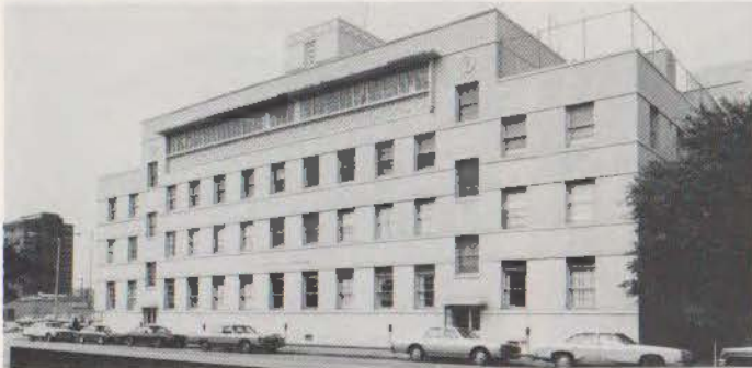
St. Joseph's Hospital additions, 1919 LaBranch, I. E. Loveless (Los Angeles), Maurice J. Sullivan, mid-1940s. Horizontal banding is broken by stair, which in turn pushes mass up to central element capped by strip window, all of which is ultimately "programmatically."
