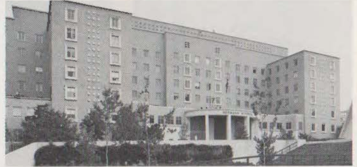
Hermann Hospital (new), Texas Medical Center, Kenneth Franzheim and Hedrick & Lindsley, 1945. One can imagine different "facade studies" to pattern the simple mass.
