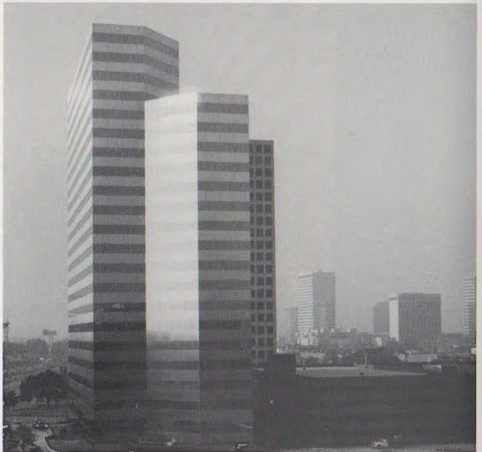
3D/International Tower, by 3D/International, for Gerald D. Hines Interests. Setbacks create extra premium spaces in 22-level tower of stainless steel and reflective glass.
