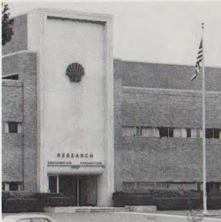
Shell Oil Co. Production & Exploration Research Bldg., 3737 Bellaire Blvd., Austin Co., 1945-47. A big theme of the 1940s: the contrast of horizontal and vertical.
