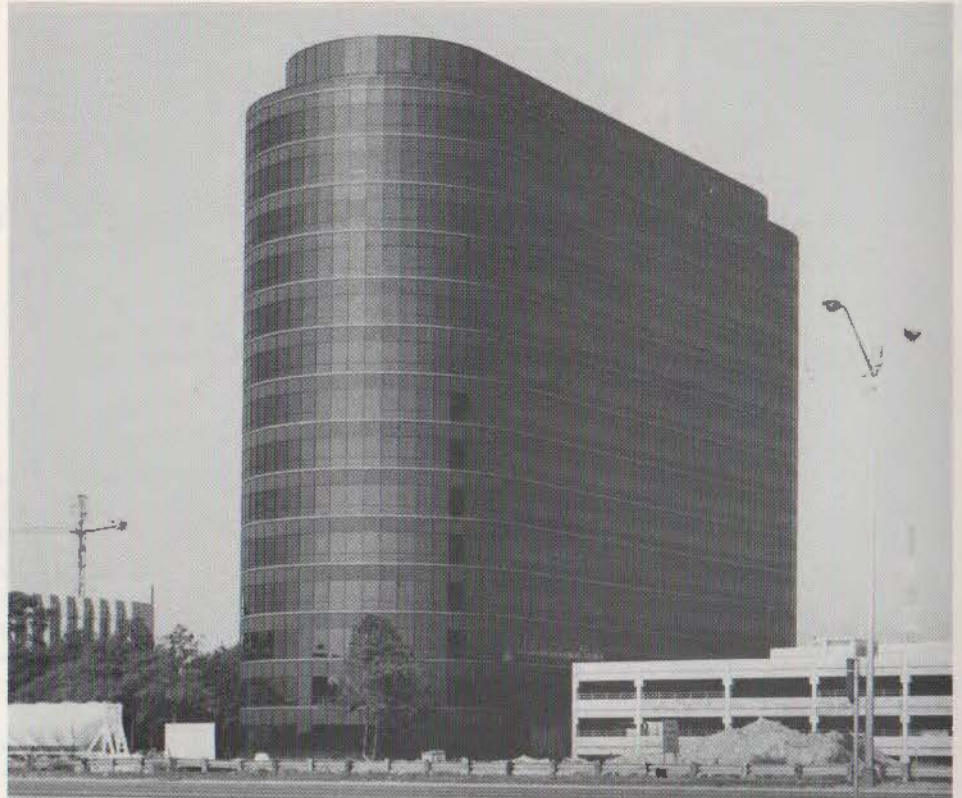
Brookhollow Central Two, by 3D/International, for P.I.C. Realty Corp. Oval configuration provides panoramic view.
