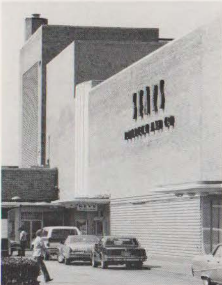
Sears Roebuck & Co., 6800 Harrisburg, Kenneth Franzheim, 1947. Raked brick joints emphasize horizontal lines, even with a stepped mass build-up.
