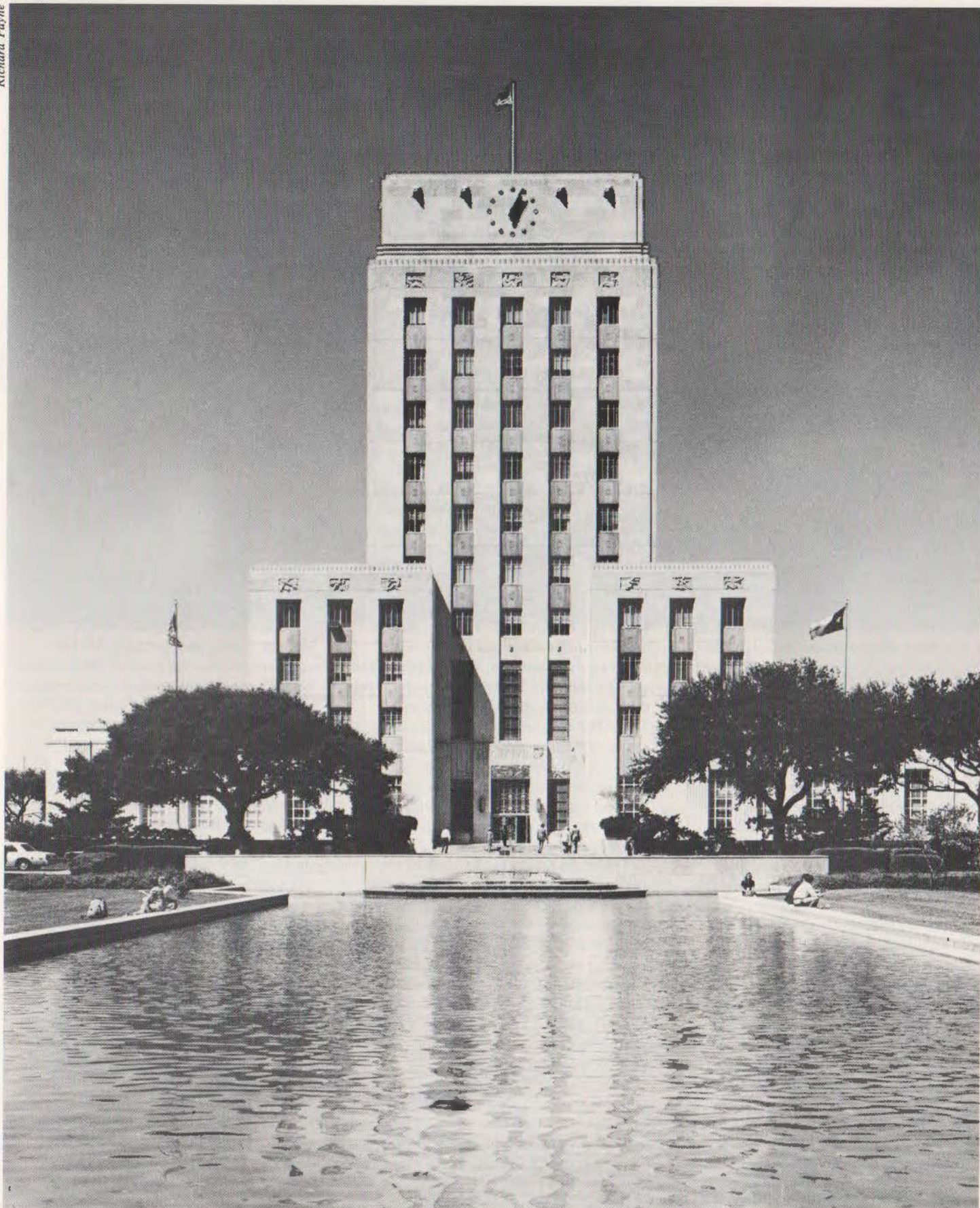
FACING PAGE: The "ordered space at Rice University" as perceived from the central quadrangle facing Lovett Hall (Cram, Goodhue & Ferguson, 1910). ABOVE: Houston City Hall, with its reflecting pool and mid-day visitors (Joseph Finger, 1939).
