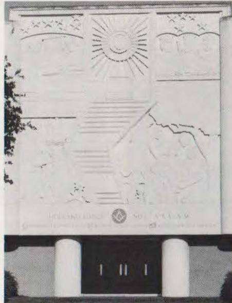
Holland Lodge #1, Masonic Temple, 4911 Montrose Blvd., Milton McGinty, 1953. Iconography dominates the architecture.
