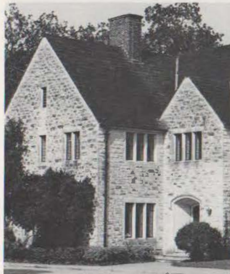
St. John's School (North Campus), 2401 Claremont Lane, by Hiram A. Salisbury, 1946-47. Country Cotswald a la Medieval/Suburbia in the manner appropriate for an Episcopal School.
