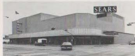
Sears Roebuck & Co., 4201 S. Main, Nimmmons, Carr & Wright (Chicago) and Alfred C. Finn, 1939. Sheathing covers the existing building; massing is all that remains. Compare this one with the other Sears stores.
