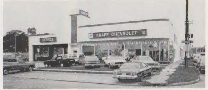
Knapp Chevrolet, 815 N. Houston Ave., R. Newell Waters and E. Kelly Gaffney, 1941. Streamlined, with slight International Style overtones, such as the "dissolving" corner.
