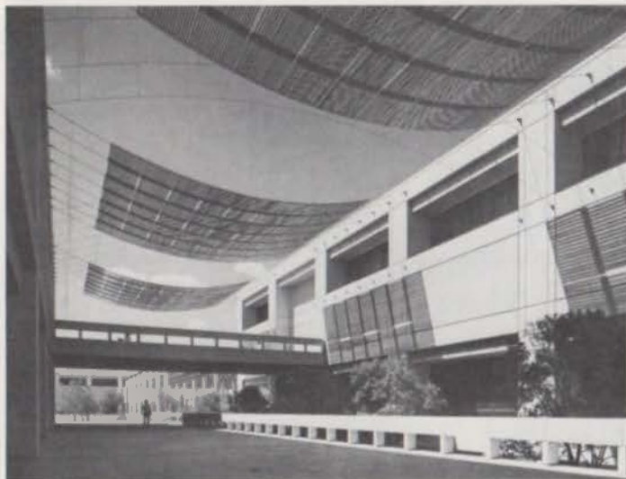
UTSA, by Rick Gardner. Architects: Ford, Powell & Carson and Bartlett Cocke & Associates.
