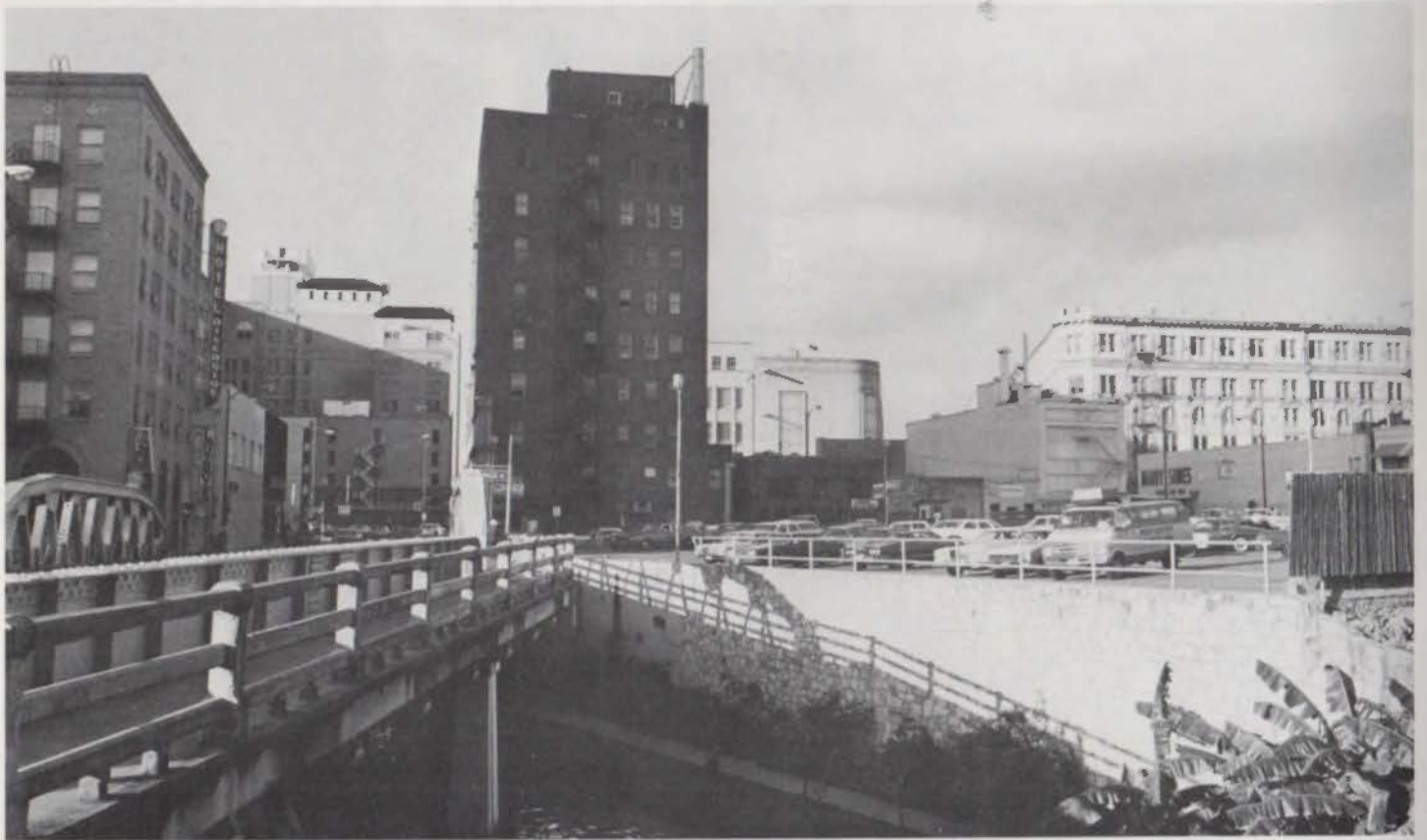
St. Mary's Street Bridge, by Judy Bankhead.
