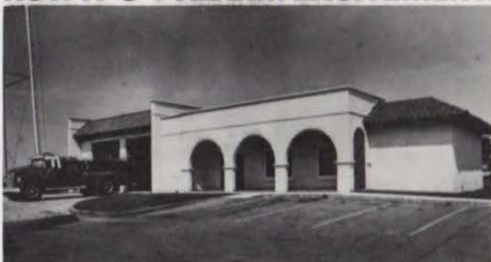
This Webb Co. Fire Station, recently completed in Laredo, Texas, was designed by Jack Rice Turner and built by the County Manpower Program.
