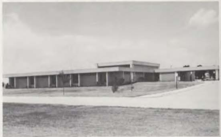
Mid-Cities Clinic viewed from Great Southwest General Hospital, Grand Prairie. Clerestory-lit waiting room.
