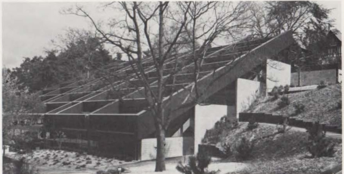
SALANTER-AKIBA-RIVERDALE ACADEMY—RIVERDALE, NEW YORK. Owner: Salanter-Akiba-Riverdale Academy. Architect: Caudill Rowlett Scott, Houston. Contractor: Miller & Raved, New York, New York.
