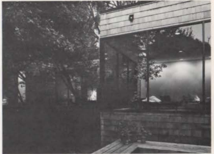
ADDITIONS & ALTERATIONS TO RESIDENCE—FORT WORTH. Owner: James Foy. Architect: Emery Young Associates, Fort Worth. Contractor: Russell A. Gill, Fort Worth.
