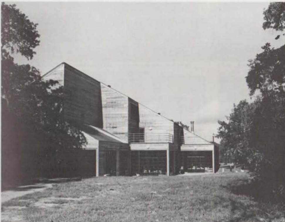
CAMP ALLEN EPISCOPAL CAMPS AND CONFERENCE CENTER — WALLER/GRIMES CO. Owner: The Episcopal Diocese of Texas. Architect: Charles Tapley & Associates, Houston. Contractors: Sentry Construction, Bryan; Bradley/Raus, Inc. and Brook Construction, Houston.
