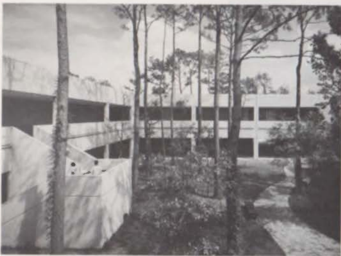
OAK VILLAGE MIDDLE SCHOOL — HOUSTON. Owner: North Forest Independent School District. Architect: McKittrick, Drennan, Richardson and Wallace, Houston. Contractor: R.M. Mayfield & Co., Houston.
