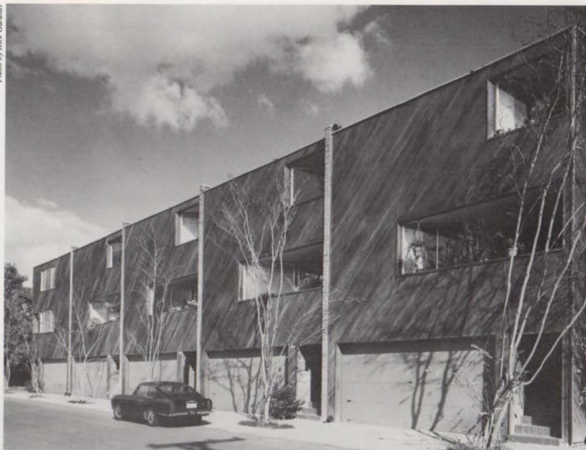
GRAUSTARK TOWNHOUSES — HOUSTON. Owner: Montrose Properties. Architect: Richard Fitzgerald & Associates, Houston. Contractor: Landmark Construction Company, Houston.
