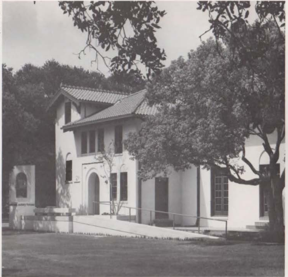
RENOVATION OF THE AUTRY HOUSE — HOUSTON. Owner: Episcopal Diocese of Texas. Architect: Bailey and Belanger, Houston. Contractor: Versi Craft, Inc., Houston.
