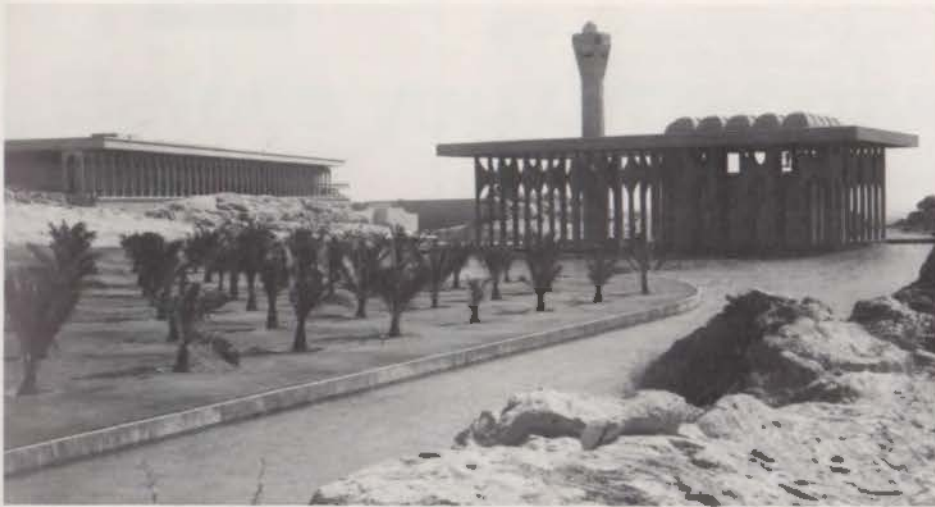
UNIVERSITY OF PETROLEUM AND MINERALS — DHAHRAN, SAUDI ARABIA. Owner: Ministry of Petroleum and Mineral Resources. Architect: Caudill Rowlett Scott. Contractors: Taisei-Jindan, Tokyo, Japan and The Consolidated Contractors Co. S.A.L., Beirut, Lebanon.
