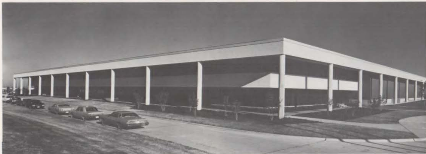
Forney Engineering Plant and Office Bldg. - Carrollton
