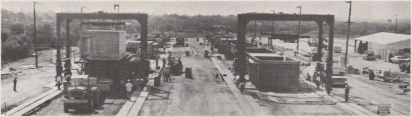
Eight units daily moved through the casting yard assembly line.
