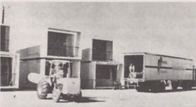
Carpeting delivered to front door of each unit.
