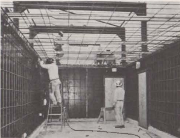
Wall and ceiling steel reinforcement in position in form.
