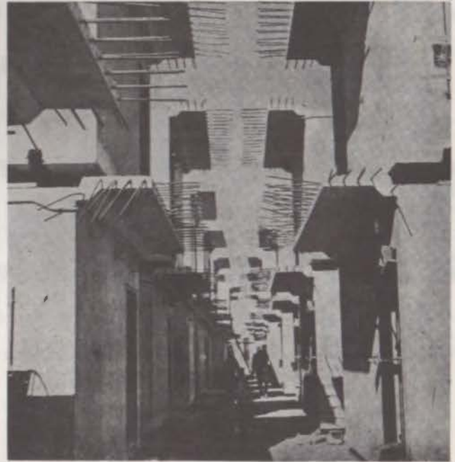
Concrete modules stacked in place at jobsite.
