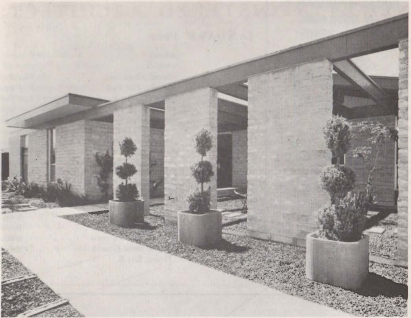
Home of Martin Meisel of Pellati and Meisel, A.I.A., El Paso . . . built with Atlas 8 x 4 x 16 tan Mission Masonry
