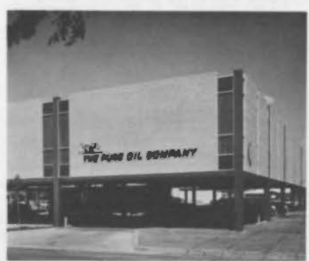
The Pure Oil Co. (Limestone Brick) — Midland, Texas Architects: Pierce, Norris, Pace — Midland, Texas
