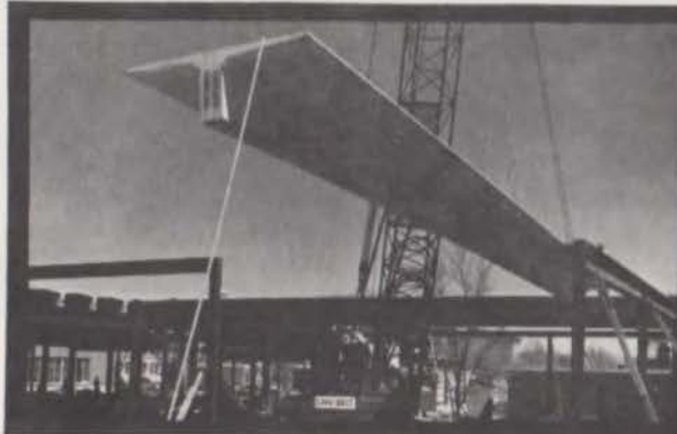
Single Tee Prestressed Unit, Student Center, West Texas State College, Canyon, Texas
