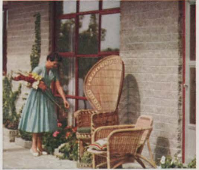
Living concrete in integrally colored 4"-high split block
