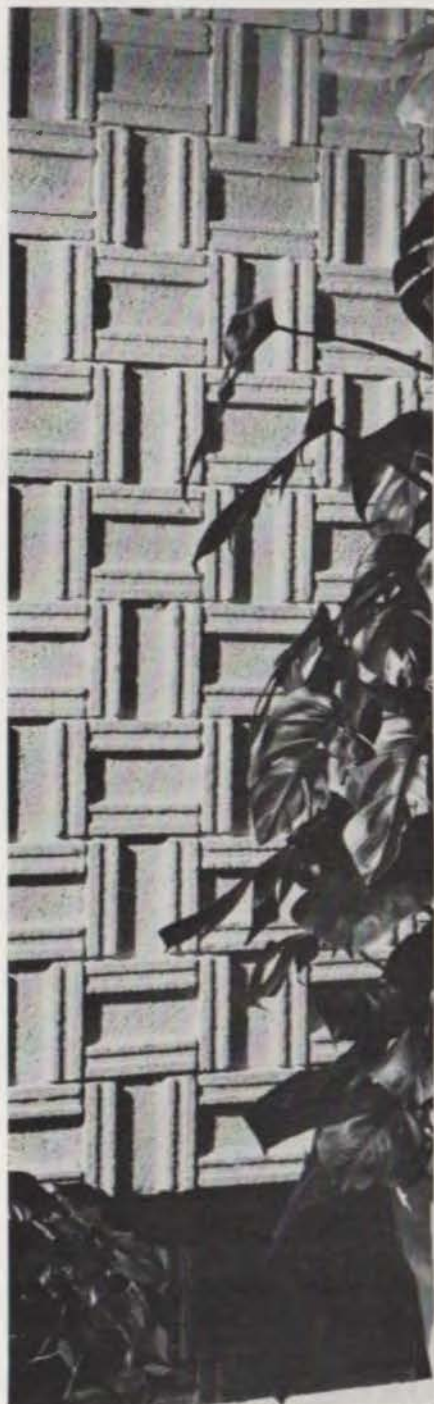
Ends of concrete block exhibit an eye-catching pattern, illustrating the flexibility of concrete masonry interior walls.
