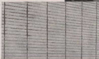
Horizontal stacking of smooth-face 2x16 inch units
