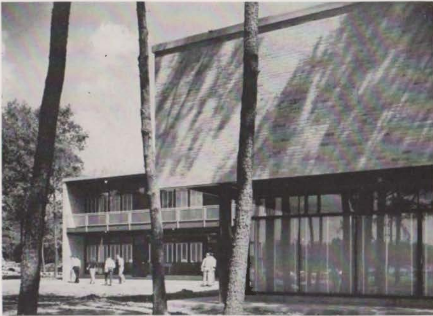
Engineering Office and Classroom Building University of Houston Houston, Texas
