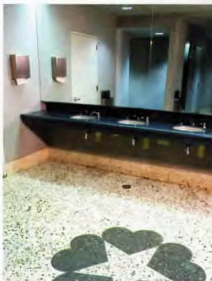
Love Field Public Restrooms
