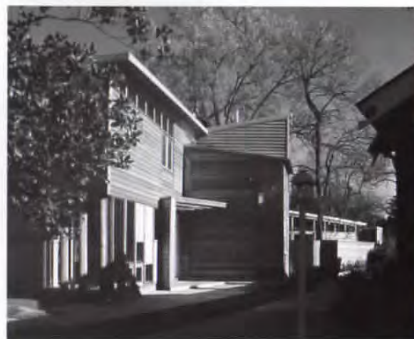
Top and above: "Elena's House" in Houston, by Pia Wortham and Joan Callis, is walled off from the surrounding neighborhood,
