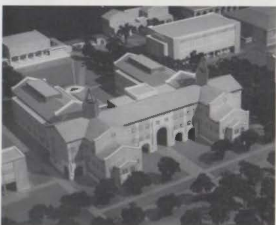
George R. Brown Hall, a 107,000-square-foot, three-story biotechnology research center at Rice University, was designed by Cambridge Seven of Boston, Mass.
