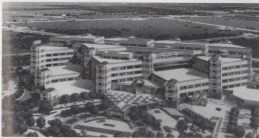
A joint venture of Houston-based 3D/International and Stone Marraccini and Patterson of San Francisco designed the new $210-million, 1.5-million-square-foot Veterans Administration Hospital (left). Site plan (below) shows the organization of patient-care wings into triangular wards for efficiency in nursing care.
