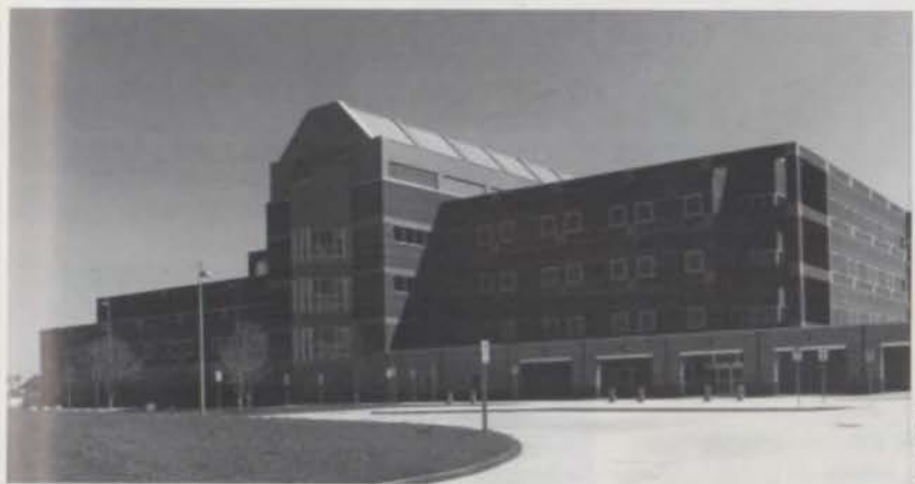
The Lyndon Baines Johnson Hospital, designed by a joint venture of Rees Associates of Texas, Inc., and Llewelyn-Davies Sahni, provides
