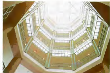
Offices are organized around a six-story rotunda.
