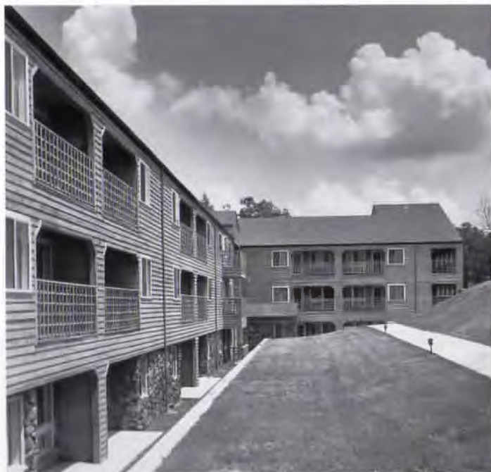
The sloping site of Pleasant Hills created problems in pedestrian and vehicular traffic for GH&F to solve, but it brought added energy to the community spaces and allowed the architects to maximize views of the surrounding forested hills.
