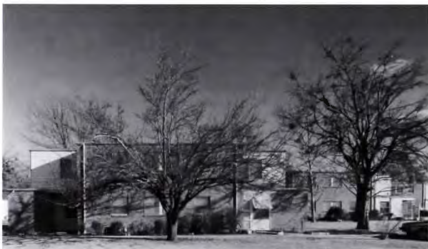
ABOVE and BELOW: The two-story apartment buildings, which show Williams's stylistic influence, have been the least altered from the original design. Only some entries have been enclosed.
