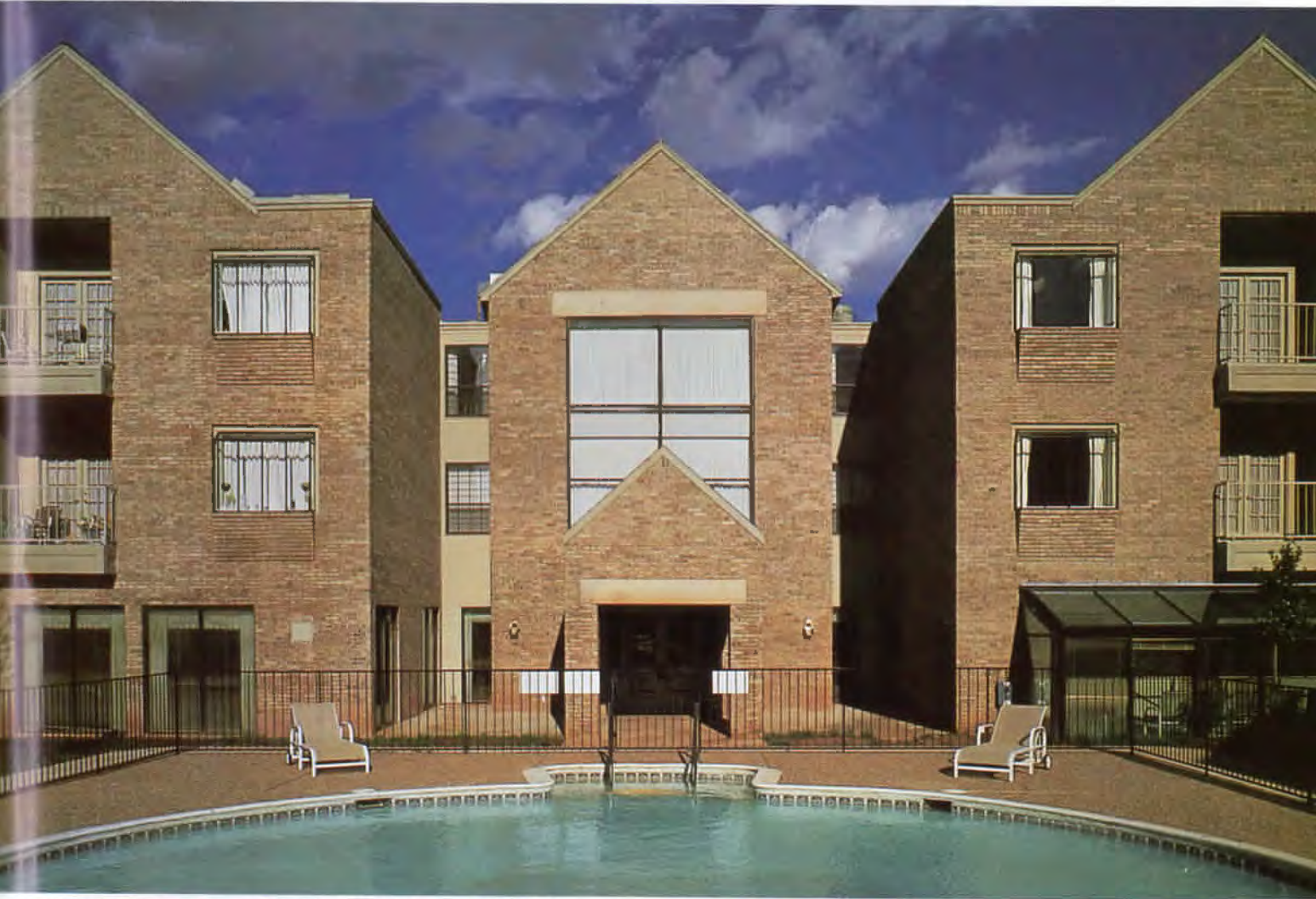
Rolling Meadows retirement center, Wichita Falls, by Good, Haas & Fulton: the west elevation of the activity center shows the use of strong, simple masses in brick as a focal point for a site uniting independent dwellings in a park-like setting with congregate-living units.
