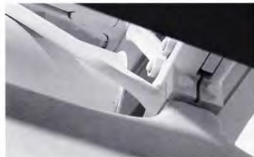
A crucial detail: the air-conditioning return-air duct tucked up above the leaves, under the glass. It removes heat before it gets down into the space below, but raises questions about the appropriateness of a glass roof for this type of building.
