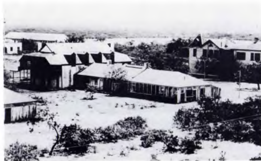
The informal early plan of Fort Ringgold Barracks, TOP, changed, until by the turn of the century it matched the standard form used throughout the West. ABOVE and BELOW: Fort Ringgold Barracks, circa 1900
