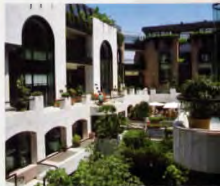
Houston Shopping Mall - utilizing thousands of square feet of thin membrane and waterproofing adhesives.
