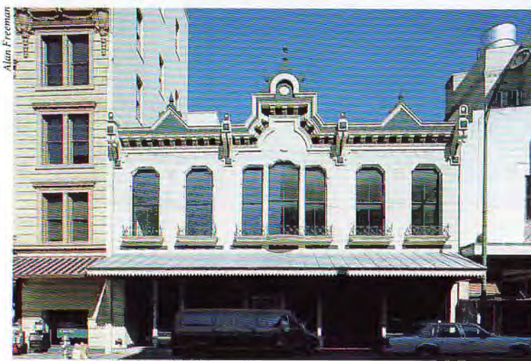
Albert Maverick Building, San Antonio
