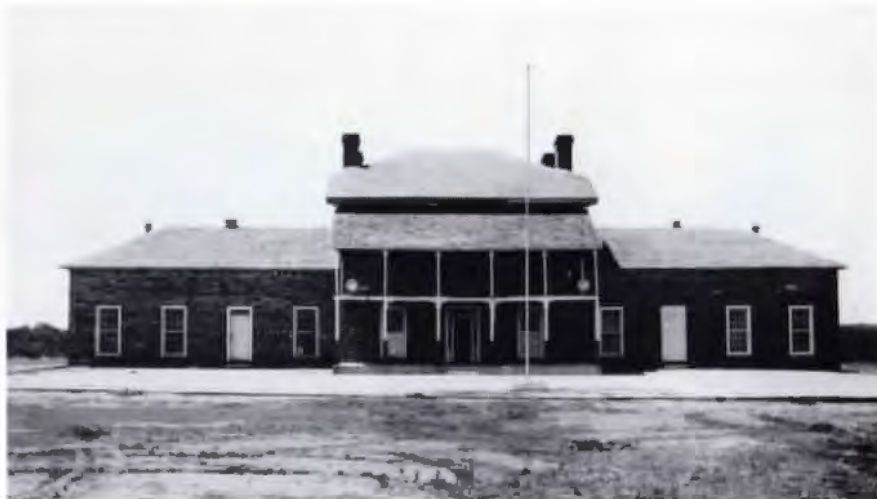
TOP: Parmenas T. Turnley made this drawing of the Turnley cottage, the prefabricated portable shelter he invented for use in the new forts of Texas, Arizona, and New Mexico. ABOVE: The hospital at Fort Richardson, built in stone as required by military regulations, has the standard two-story central block with one-story wings.
