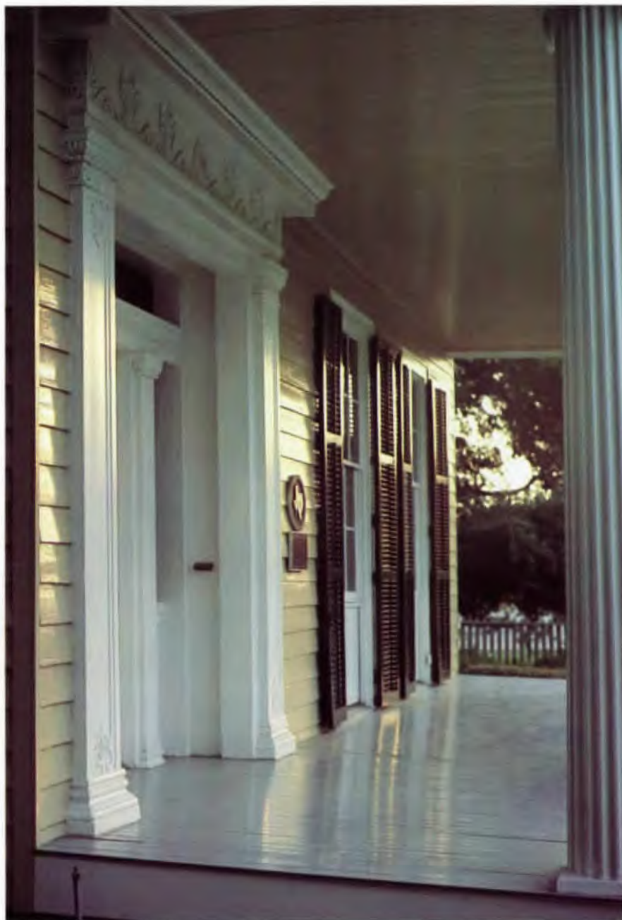
The Nichols-Rice-Cherry house was built in Houston around 1850. Its doorcase and door and the painted and grained interior details are all derived from the Lafever-Benjamin repertoire. These details represent the ultimate level of decoration reached in Texas in the antebellum period, and are the most elaborate surviving examples in the state.
