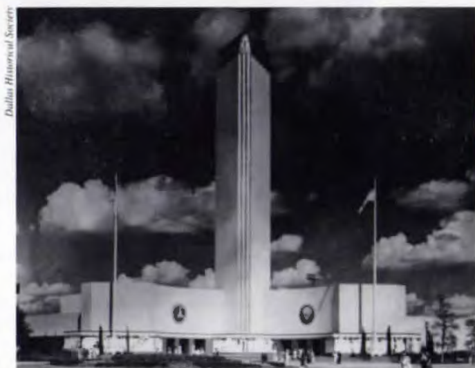
The Federal Building circa 1936.
