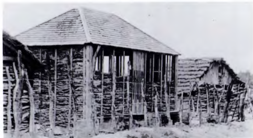
Early construction at some western forts was based on stick-and-mud structures like these Mexican-built jacales photographed circa 1890 near Fort McIntosh. Except as noted, historic photographs and drawings are provided courtesy Barker Texas History Center.
