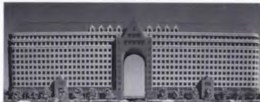
Providence Towers in Farmers Branch, 1986, by Morris/Aubry Architects
