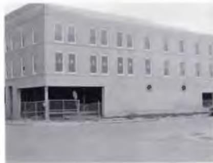
Cody Building —Fort Worth Built 1910 Renovated 1986 Owner: Aubrey Webb Architect: Daneshiou-Shum Inc. Const. Co.: Thomason & Newman
