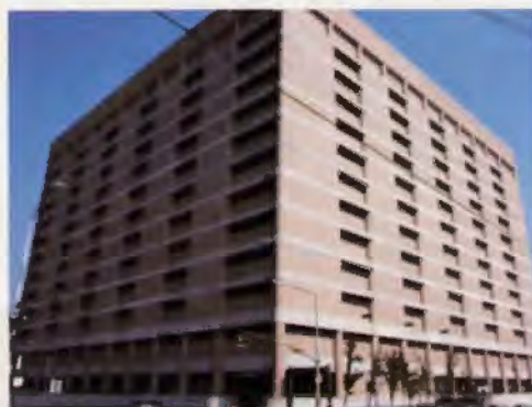
Southern Texas Correctional Facility - over 100,000 square feet of sanitary commercial flooring.
