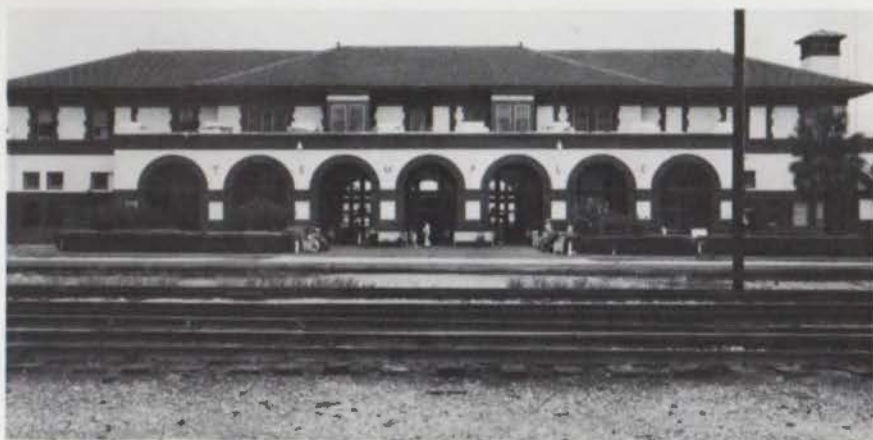
The Temple depot, once a community focal point, also houses Amtrak ticket offices.
