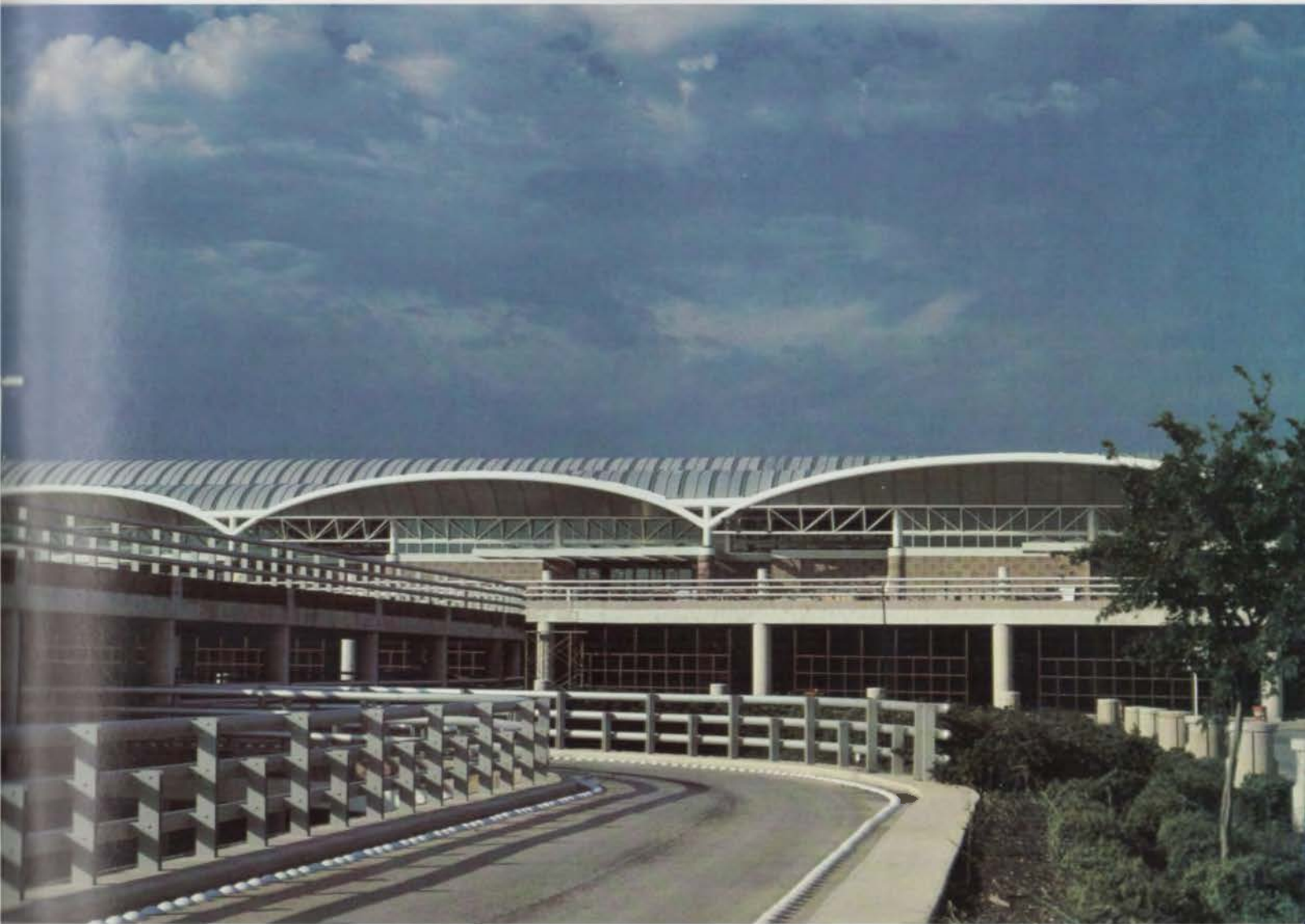
Clever use of finish materials and spatial orientation keep this terminal more on the side of efficiency than monumentality.
