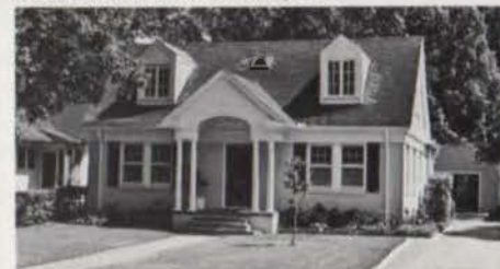
Heineman House renovation
