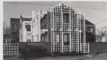
1940s house renovation by SIR
