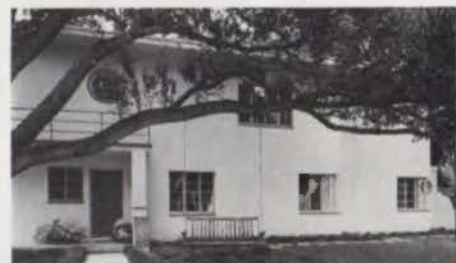
1930s house renovation by Cannady
