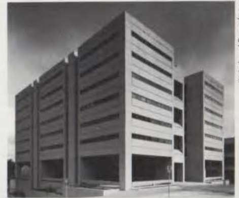
Travis County Jail
