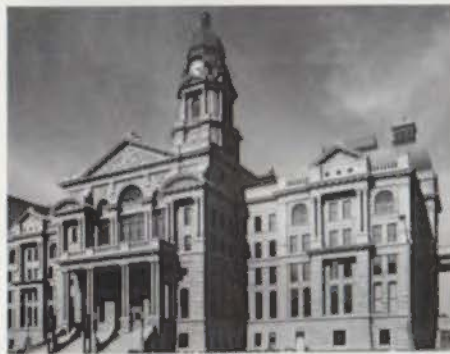
Tarrant County Courthouse
