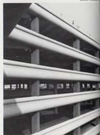
Detail of parking structure at Dallas Galleria. Straightforward, yet not without a certain elegance, this is a parking garage that looks like a parking garage. Architect: Hellmuth, Obata & Kassabaum, Dallas.
