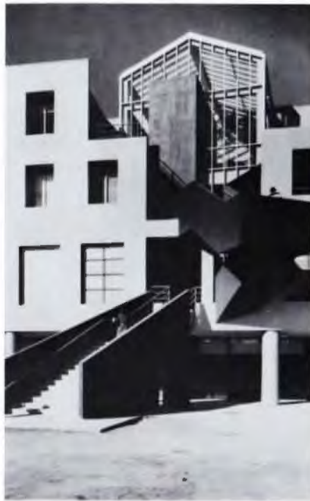
Fritz B. Burns Buildings by Frank Gehry, Loyola University Law School, Los Angeles.
