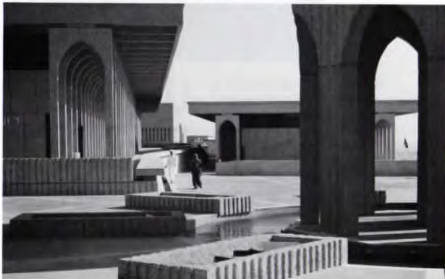
CRS' University of Petroleum and Minerals, Saudi Arabia: a product of 17 years of interchange with the users, one key to "fourth-stage" architecture.
